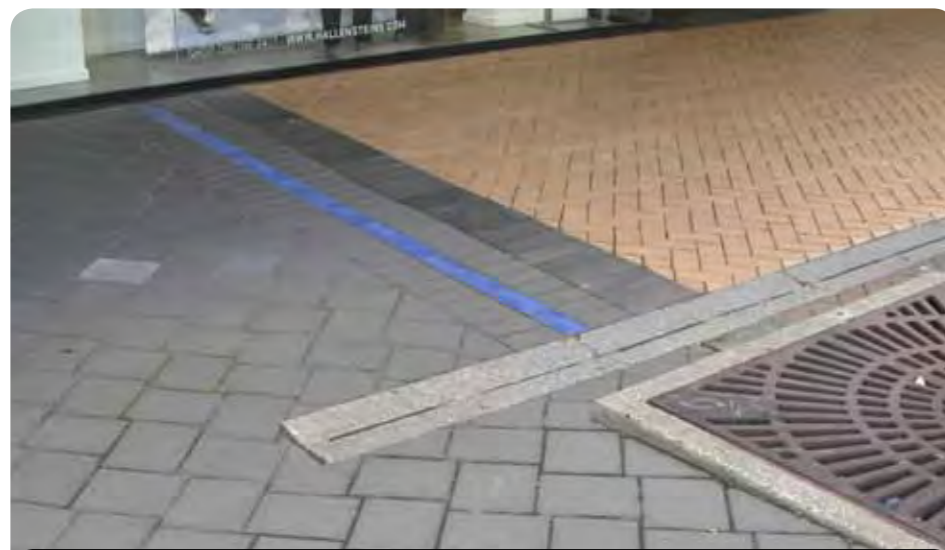
Visual clutter created when surfacing materials meet
