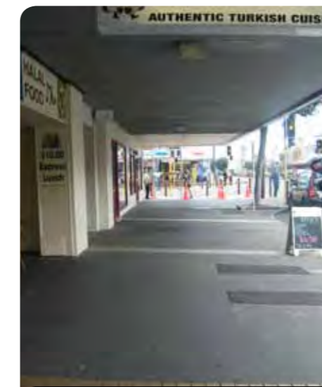
Asphalt footpath with paving strips
