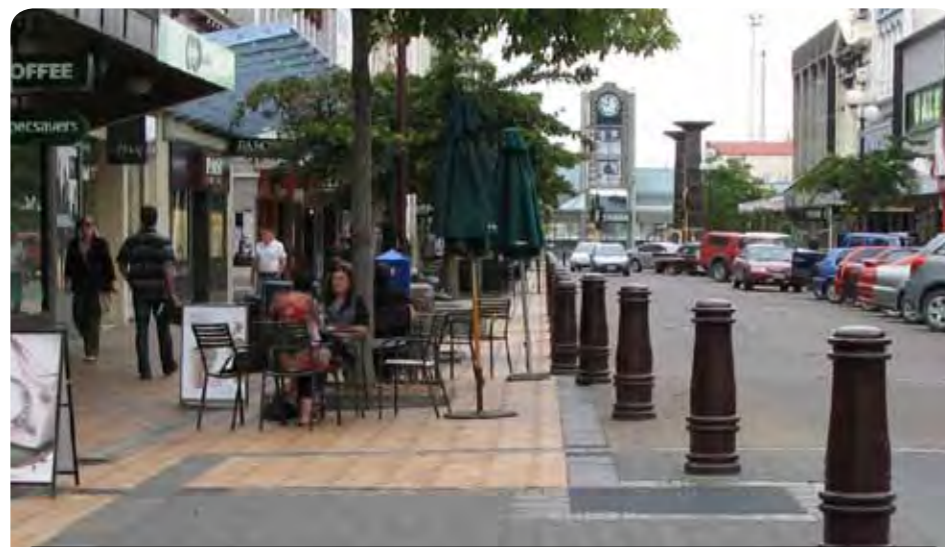
Large bollards on Esk Street to separate traffic and pedestrian
