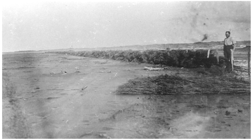
Early attempts at erosion control with the construction of brush fences to catch the sand - 1924
