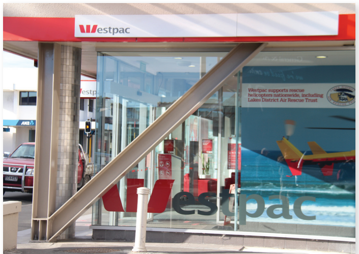
Westpac bank building on the Kelvin/Spey Street corner of the CBD showing an example of earthquake strengthening.
