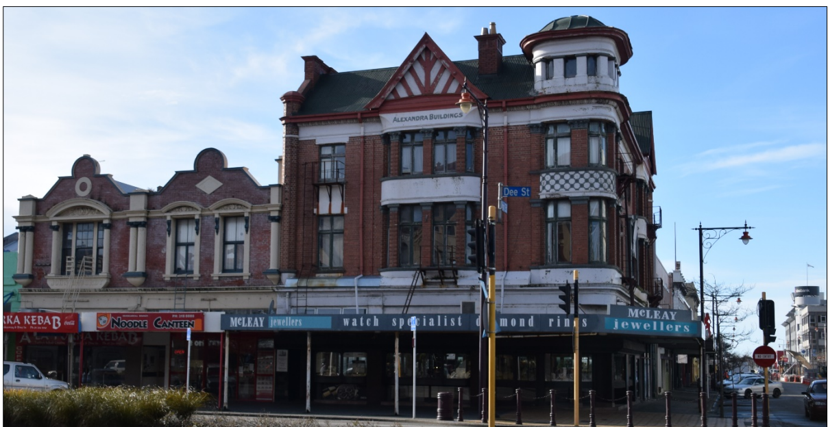
Figure 8: 83 Dee Street/2 Don Street – the Alexandra Buildings constructed c.1901 to a design by CJ Brodrick in Arts and Crafts style.
