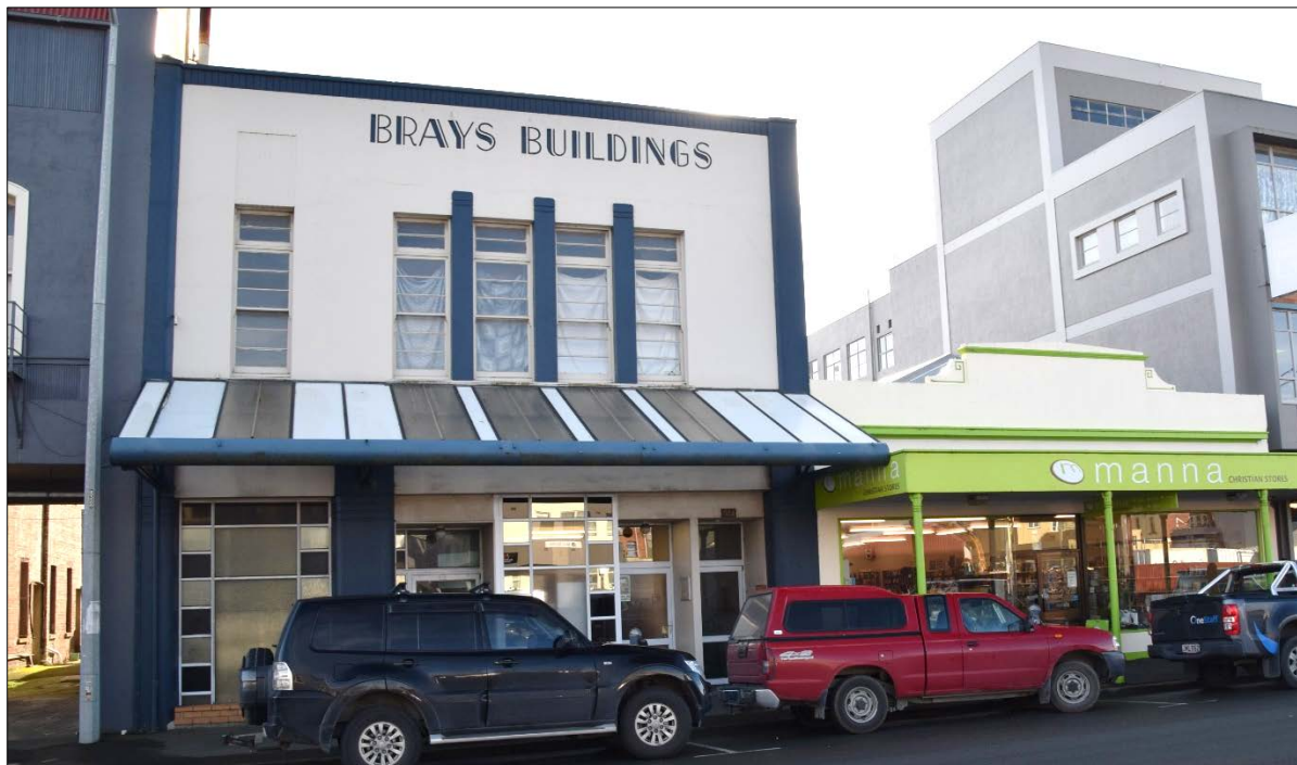
Figure 9: 88 Spey Street – Brays Buildings constructed c.1930 as auction houses for T MacGregor, with simple Art Deco vertical detailing.
