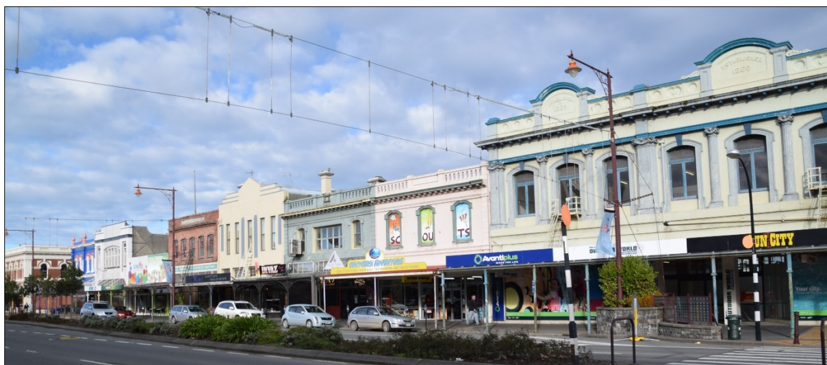
Figure 18: Tier 2 buildings along Tay Street incorporating Victorian, Edwardian and Art Deco commercial design styles.
