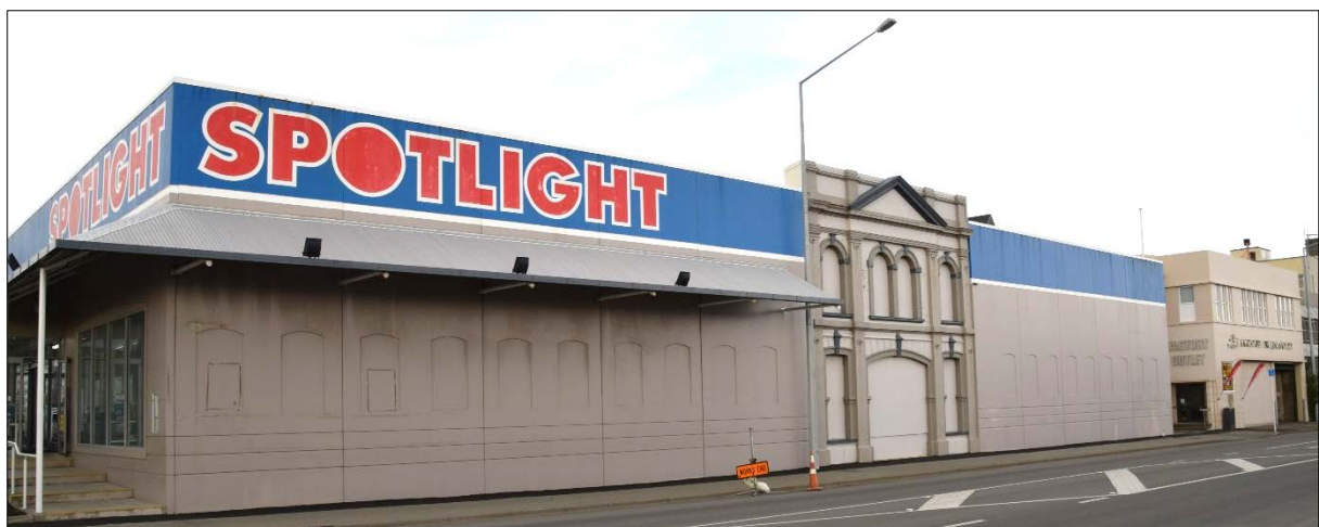
Figure 25: 33 Leven Street – the rear elevation of the Spotlight building with the remnant of the former Macaulay's Building façade in the centre.
