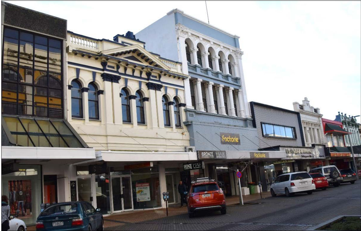
Figure 19: Tier 2 (and 1) buildings along Esk Street incorporating classical Victorian and Edwardian commercial design styles.
