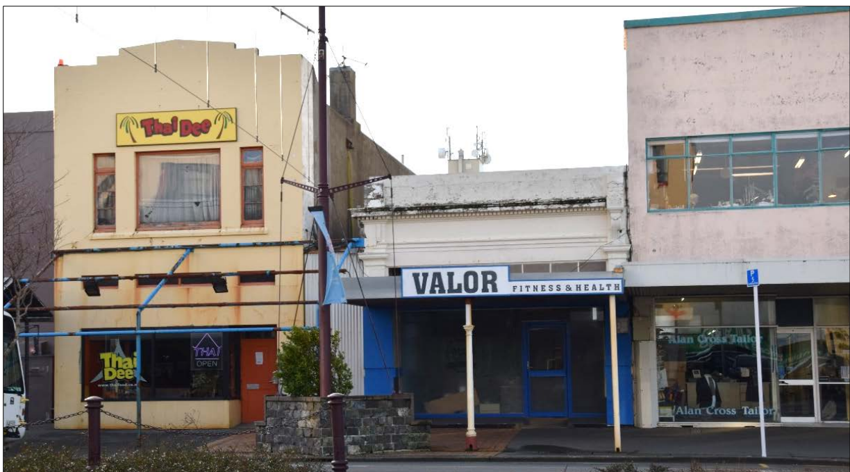
Figure 24: 7 and 9 Dee Street (Thai Dee and Valor Fitness) recommended for removal from the list of Site of Local Significant due to their low streetscape contribution.
