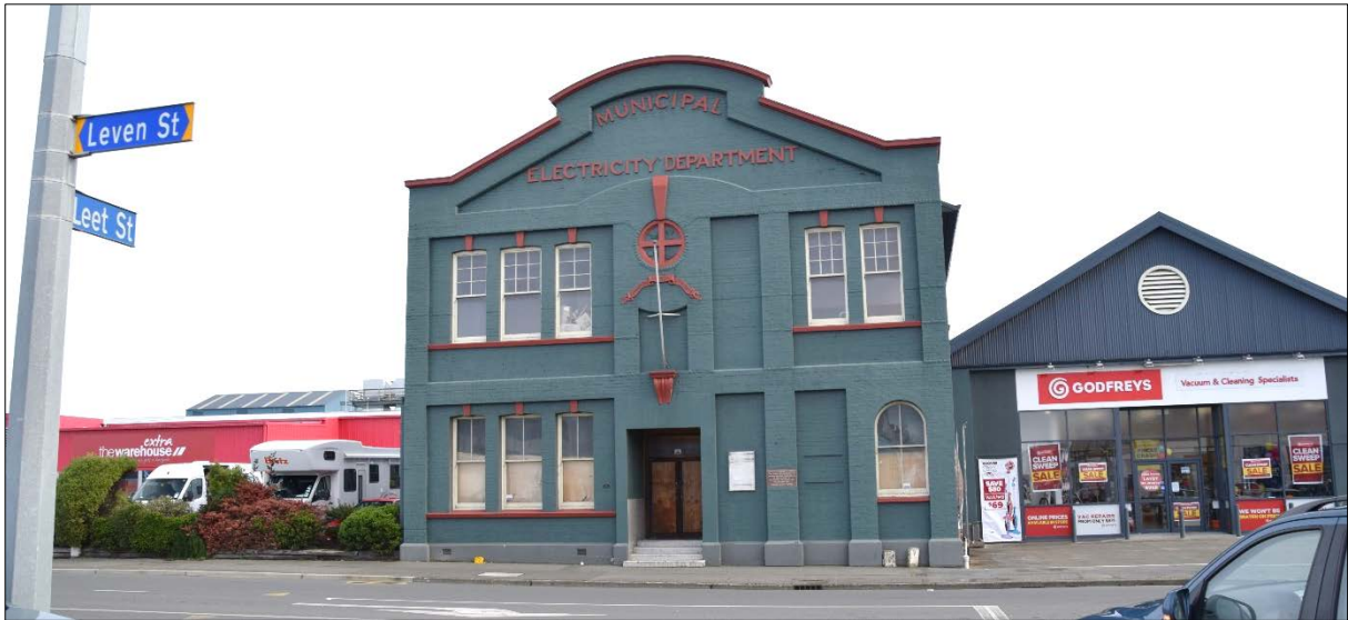
Figure 16: Tier 1 buildings - The Municipal Electricity Building and Tram Barn at 90 Leven Street.
