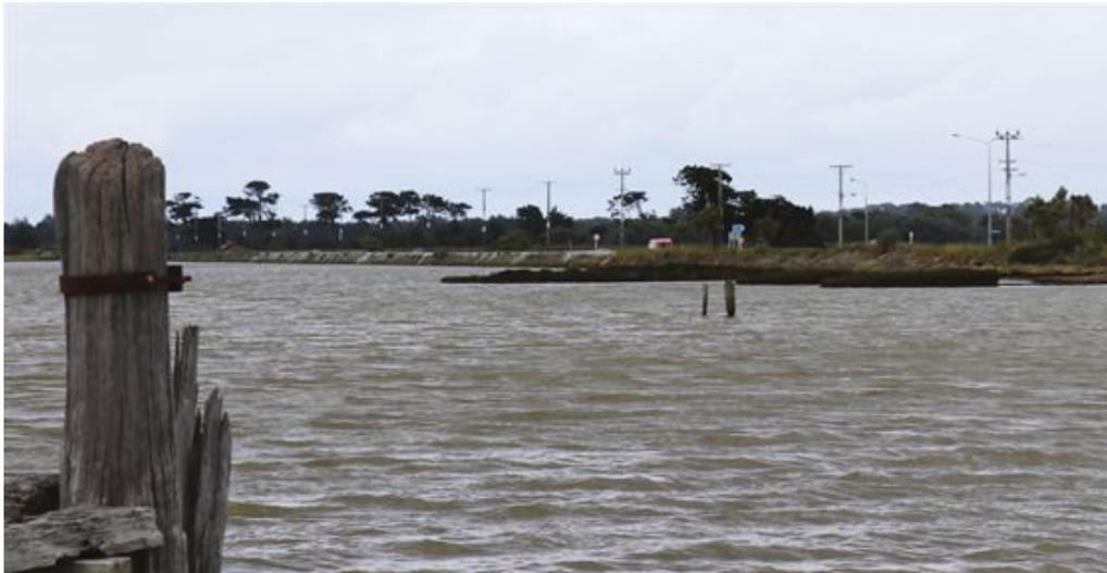
The Stead Street stopbank was constructed in 1910, and protects the Invercargill airport, Stead Street, and parts of the residential area of Otatara from tidal flooding. It was overtopped in March 2016 due to a very high tide amplified by a storm surge. With predicted sea level rise the risk of overtopping will increase in the future. This project intends to reconstruct the stopbank to current standards, and to raise it to protect against the expected 2100 storm tide level.
