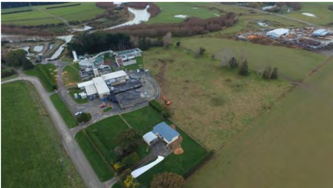
Existing plant as of June 2016
