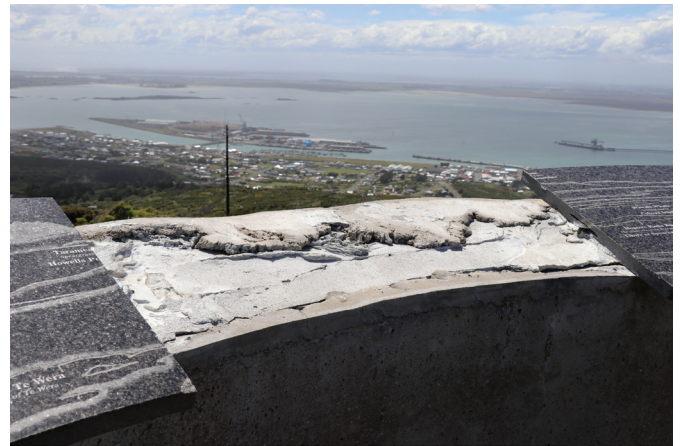
The vandalised Bluff Hill Panels.
