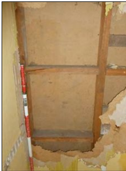
Figure 6-48. Sample area 21A with timber framing exposed (photo facing west).
