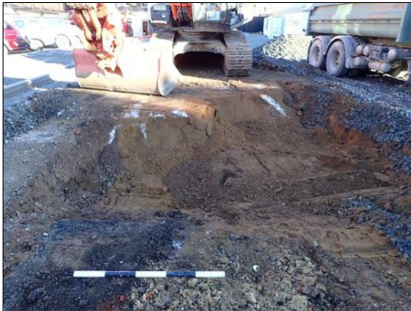
Figure 4-19. Context AS83 after excavation. Photo faces south.
