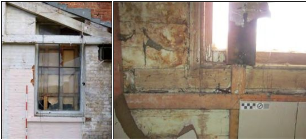
Figure 7-11. Right: photo of covered window in room 2 from exterior (photo facing south) Right: interior detail of window from Sample Area 2A (photo facing north).
