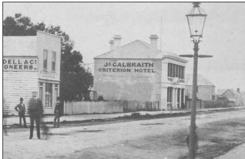
Figure 6-12. Detail of the Criterion Hotel from a photograph looking north-east along Don Street 27 .
