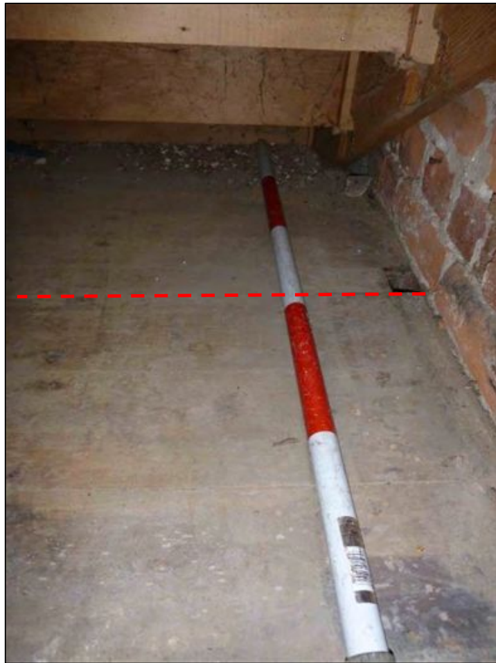
Figure 6-27. Photo of sample area 9A showing tongue-and-groove floorboards, red dashed line marks end of wider floorboards (photo facing south) (scale in 20cm increments).
