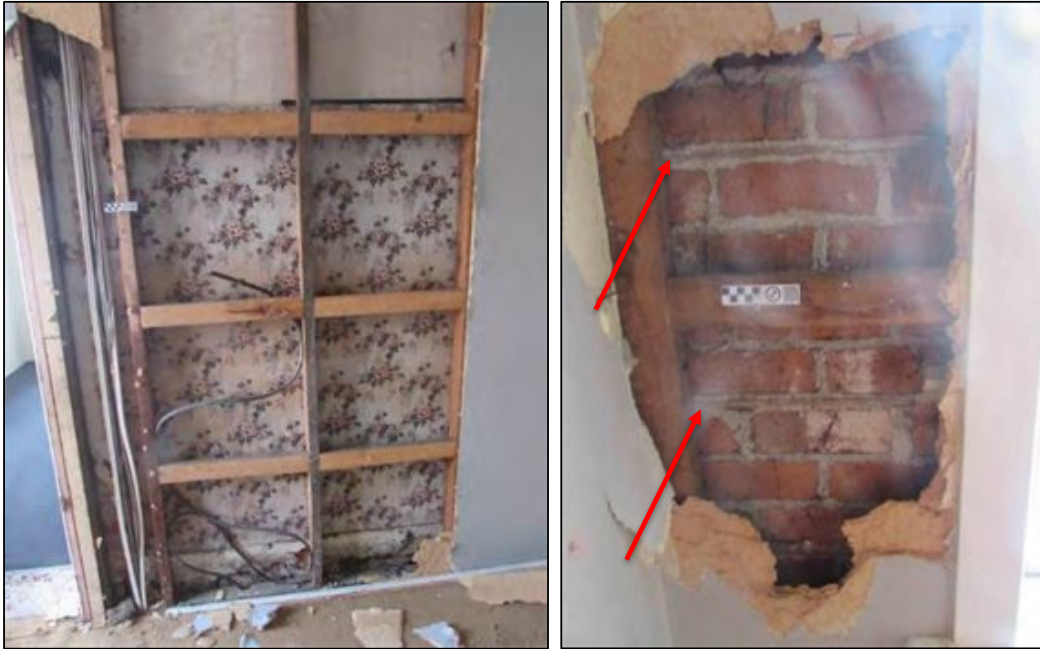
Figure 6-42. Left: photo of sample area 18A with wallpaper 1 exposed behind modern linings (photo faces west). Right: photo of brick wall exposed in sample area 18B red arrows point to planks identified between courses (photo faces south).
