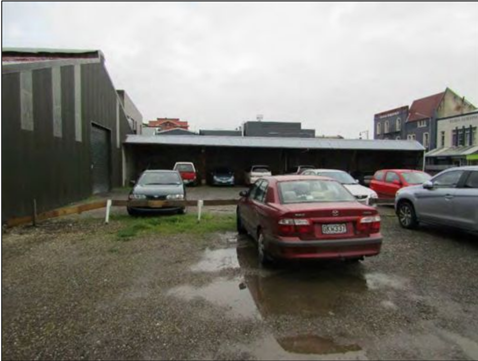
Figure 1-5. View of Sections 4 and 3 prior to the commencement of site redevelopment, with buildings on the left and car parking on the right. Photo facing west.
