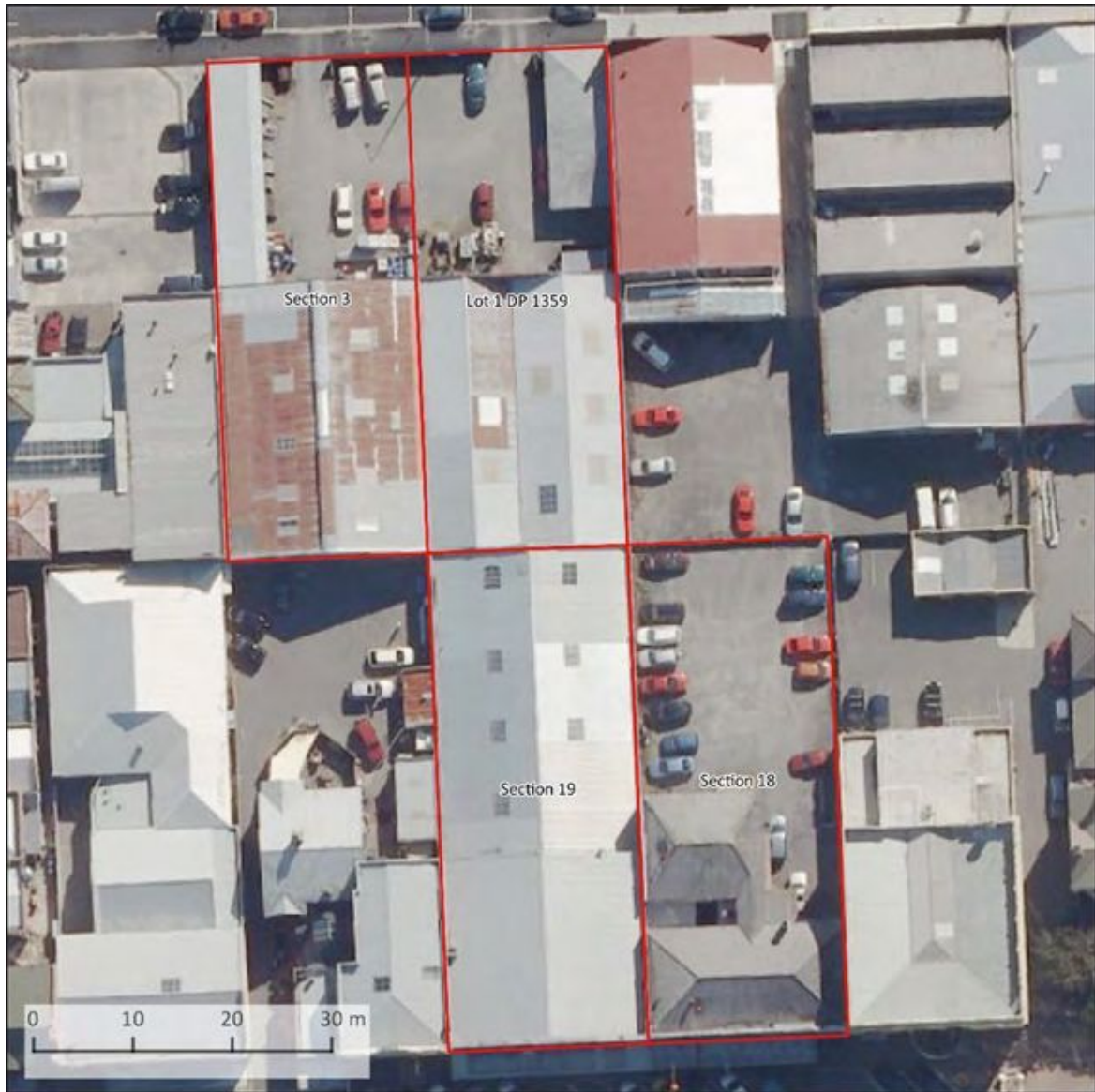
Figure 1-4. Aerial photograph showing the extent of the buildings covering the project area prior to works commencing. Aerial image courtesy of the Invercargill City Council.
