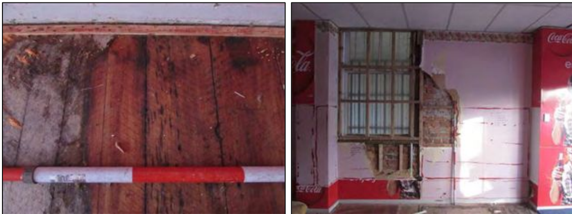
Figure 6-17. Left: photograph of Sample Area 1C showing the transition from narrow to wide floorboards (photo facing west). Right: photograph of the sash window and brickwork exposed in Sample Area 1A (photo facing east).
