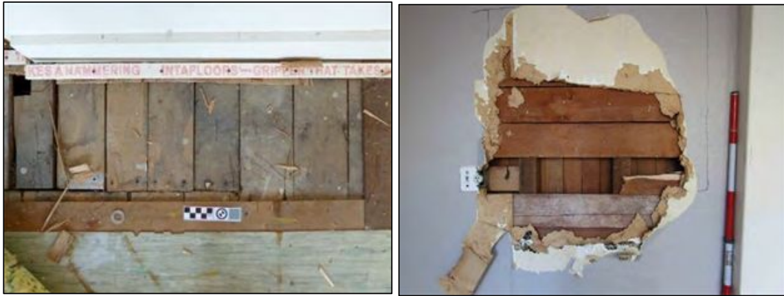
Figure 6-60. Right: sample area 24B showing area of narrow floorboards (north to top of photo). Left: photo of sample area 24A showing sarking behind modern softboard lining (photo faces north).
