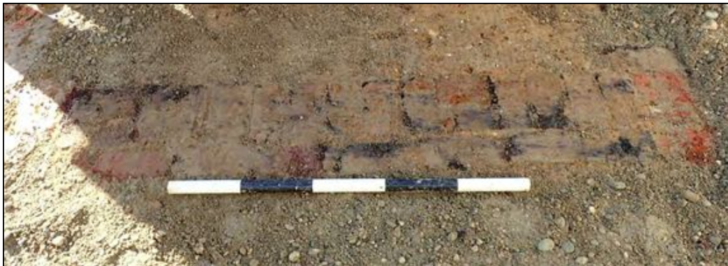
Figure 4-11. Context AS69, brick footing. Photo faces east.
