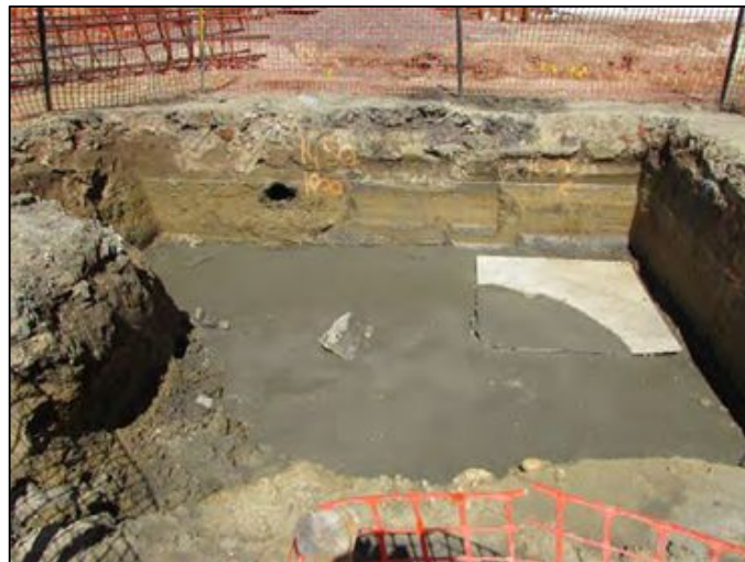
Figure 2-10 Area AF, hole area excavated for lift shaft, Photo faces south.
