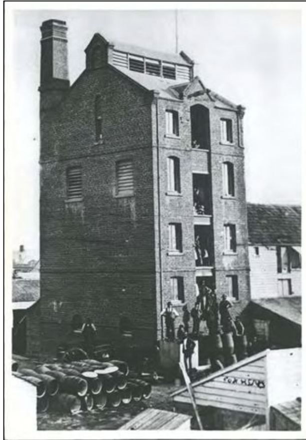
Figure 1-12. The five-storey brick building at the Black Eagle Brewery 5 , constructed circa 1874-1875.
