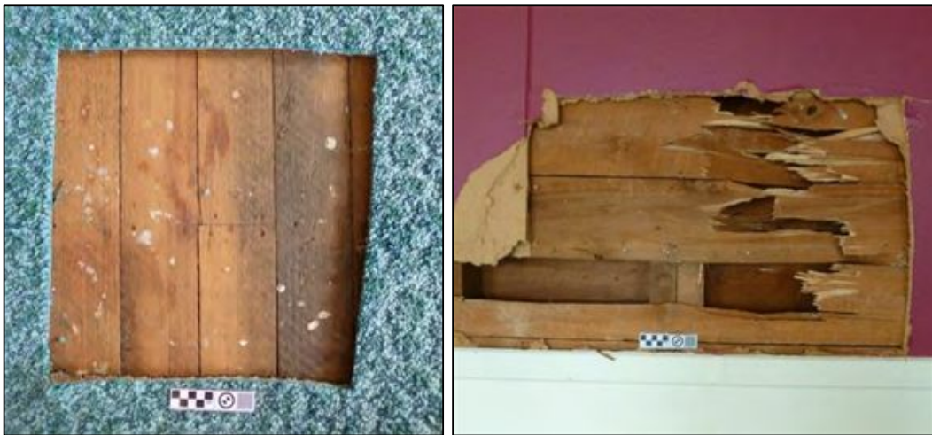
Figure 6-62. Right: sample area 25A showing tongue-and-groove floorboards (north is to right of photo). Left: sample area 25B showing sarking boards (photo faces south).
