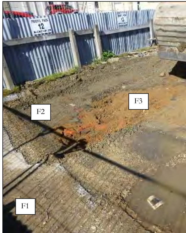
Figure 6-68. Photo showing some of the layers identified at the rear of the site during the site scrape F1 asphalt, F2 gravel, and F3 silt and gravel. Photo faces south-east.
