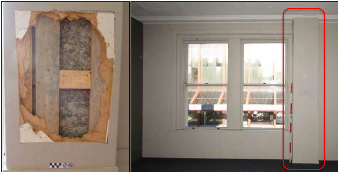
Figure 6-39. Left: Sample area 17A with concrete column exposed. Right: south wall of room 17 showing column still covered by softboard lining (photos face south).
