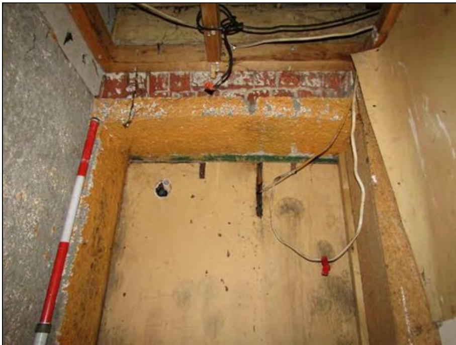
Figure 6-23. Photo of brickwork and roughcast walls identified in Room 6, scale is in 20cm increments (photo facing south).
