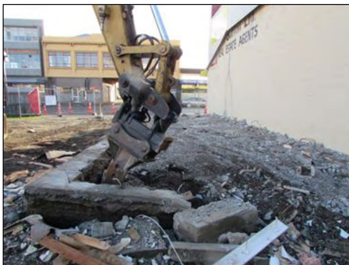
Figure 2-2. Removal of post-1900 building foundations (Area AQ). Photo faces north.
