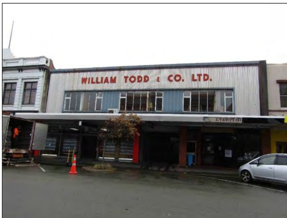
Figure 1-9. View of the William Todd & Co. in the Rialto Building on Section 19 from Don Street prior to site redevelopment; photo facing north.
