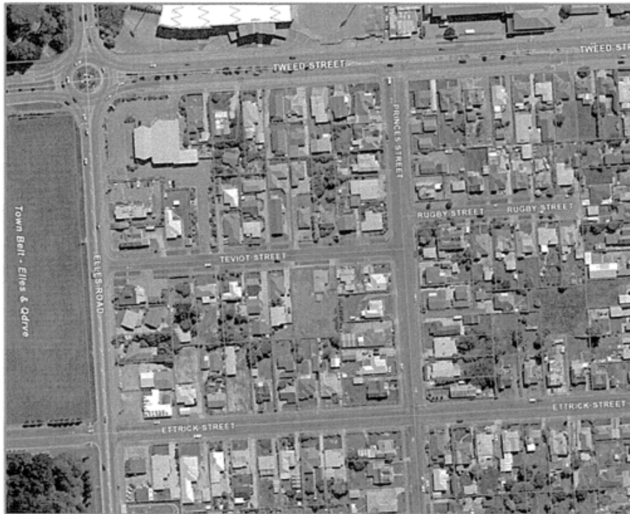
Receiving Environment – Aerial Overview
