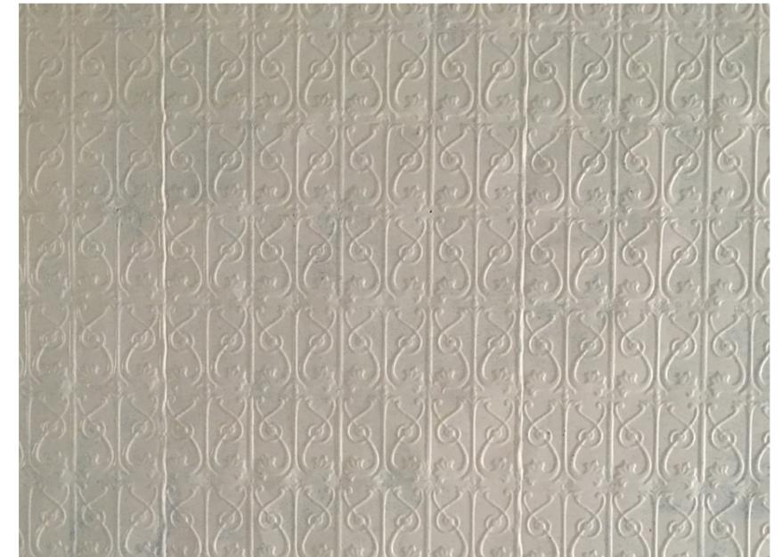
Pressed metal ceiling will be reused to clad the bar and cafe counters subject to condition.
