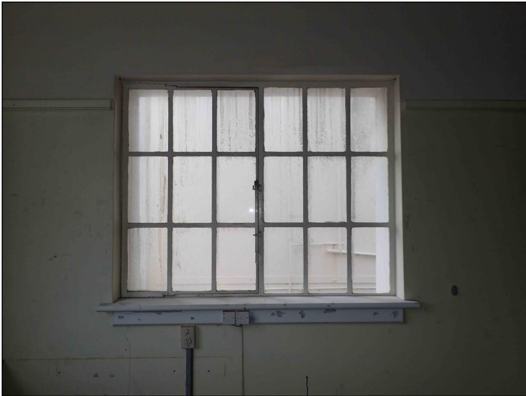
Figure 6-270. Multi-paned steel casement windows in east wall of Room 13.
