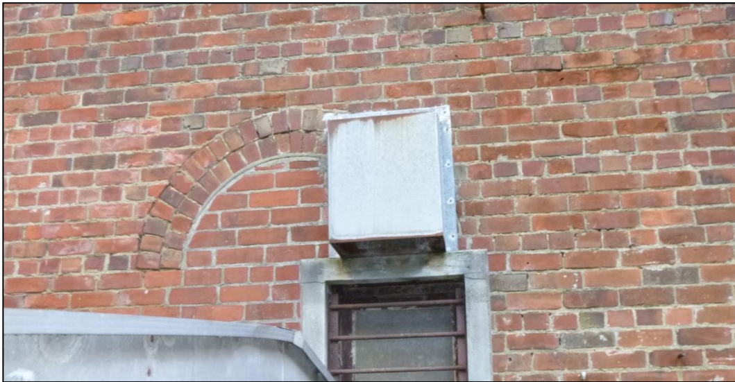
Figure 6-161. Detail of filled in window, west elevation of Martin, Maitland & Co.'s Building.
