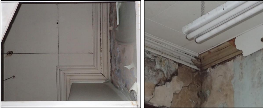
Figure 6-152. Traditional moulded cornices on the first floor of Coxhead's Building.
