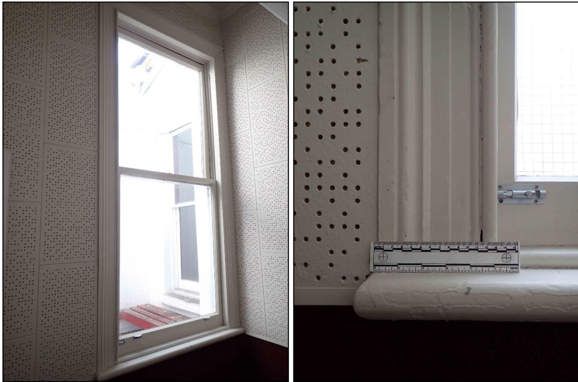
Figure 6-356. Sash window and detail of architraves.
