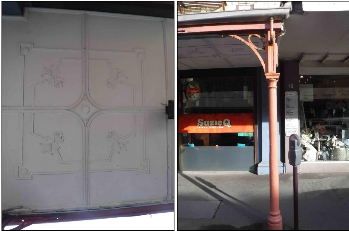
Figure 6-350. Details of fibrous plaster verandah ceiling (left) and iron posts (right).
