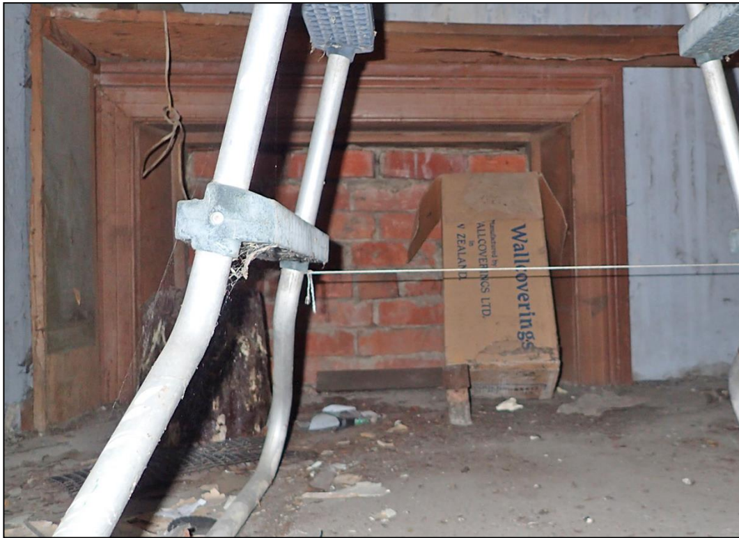
Figure 6-156. Bricked up window above Room 23 (strongroom). This indicates that the window predates both the strongroom and the upper levels of the building immediately to the west. (Lewis and Co.'s Building).
