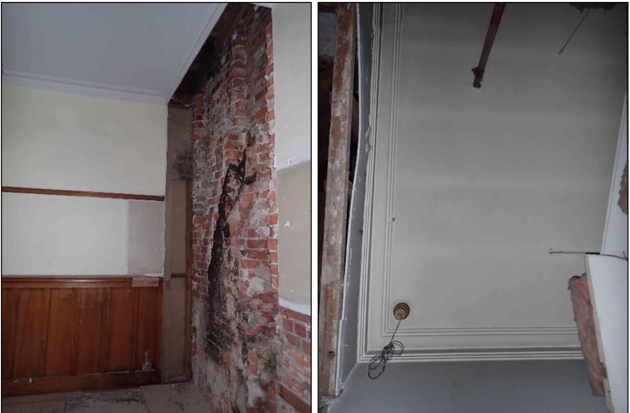
Figure 6-259. Left: Fireplace scar, wainscoting and dado rail in Room 48. Right: Cornice and original ceiling in Room 48.
