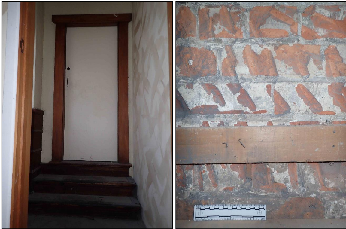
Figure 6-260. Left: wide architraves and wainscoting in Room 63. Right: scouring on bricks in Room 48.
