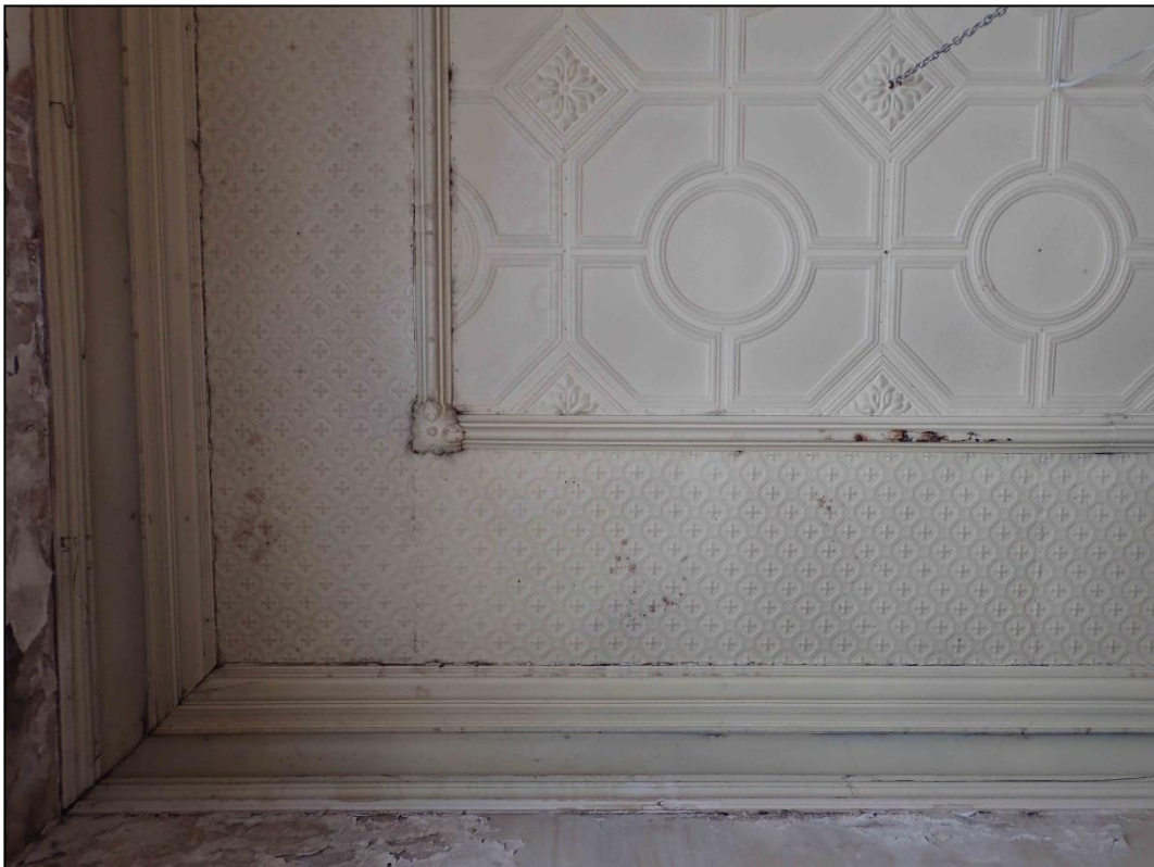
Figure 6-375. Pressed tin ceiling and moulded cornices at 48 Tay Street.
