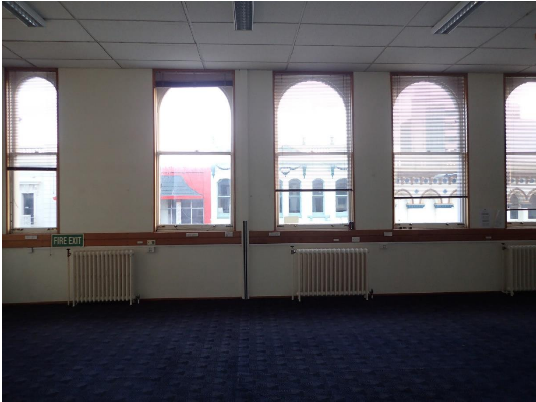
Figure 6-198. The double hung sash windows in the north wall of Room 9. Note the smaller window to the left, which is the central window in the façade.
