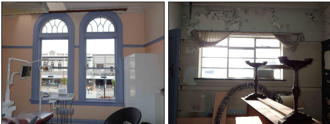
Figure 6-245. Timber sash (left) and steel fixed/awning windows (right) at 40 Tay Street.
