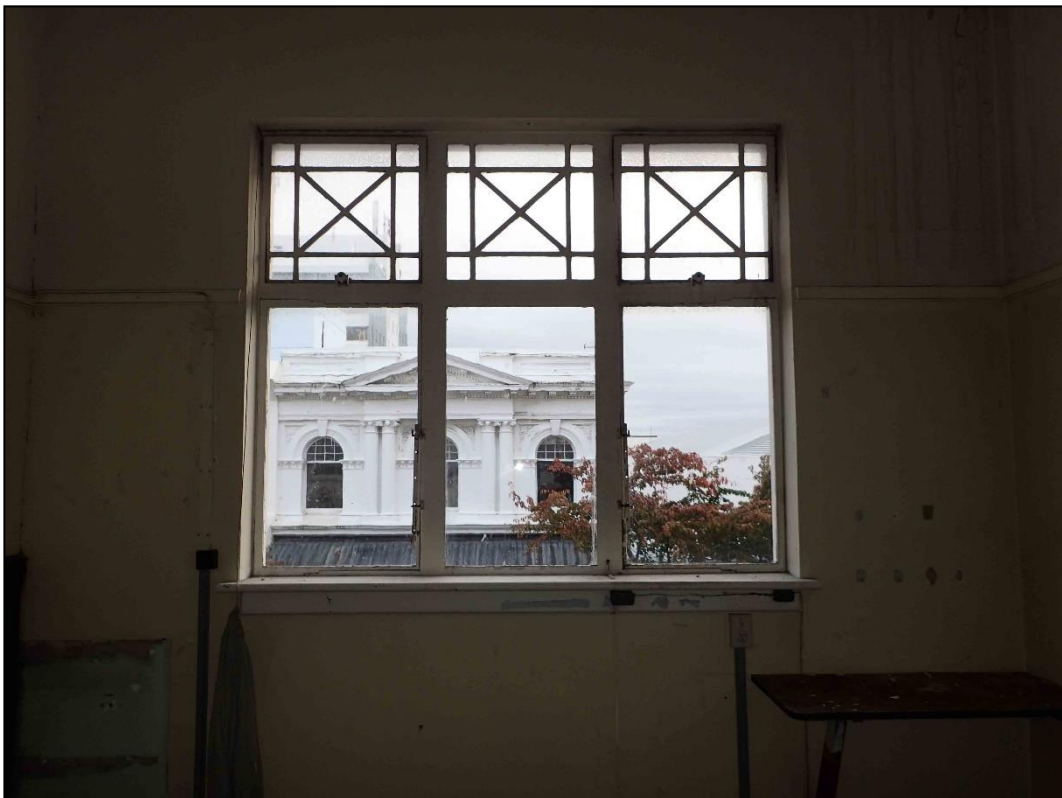
Figure 6-271. Casement windows with leadlight quarter lights in north wall of Room 12.
