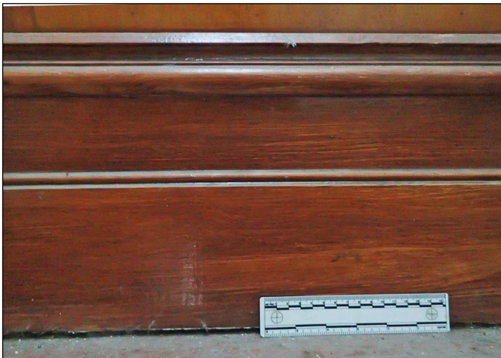
Figure 6-155. Traditional moulded skirting boards, south wall Room 20 (landing).
