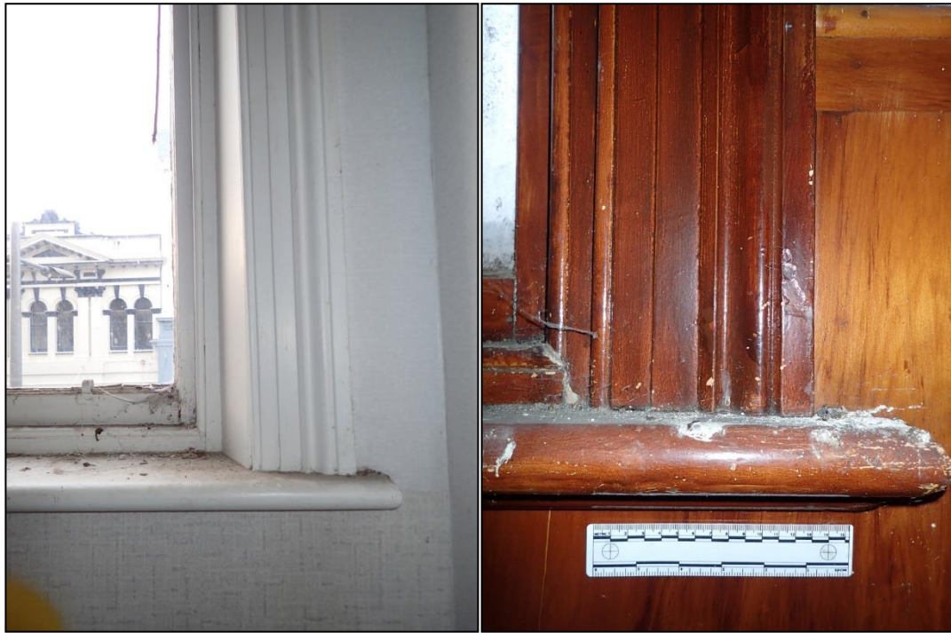
Figure 6-154. Original traditional moulded window architraves. Left: north wall of Room 21. Right. North wall of room 22.
