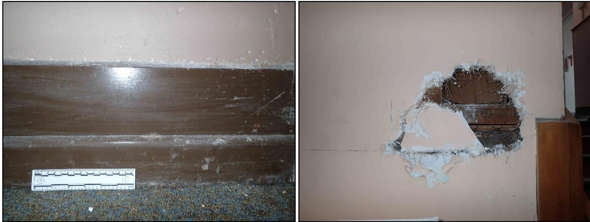
Figure 6-277. Left: detail of Art Deco skirting. Right: exposed section of fibrous plaster.
