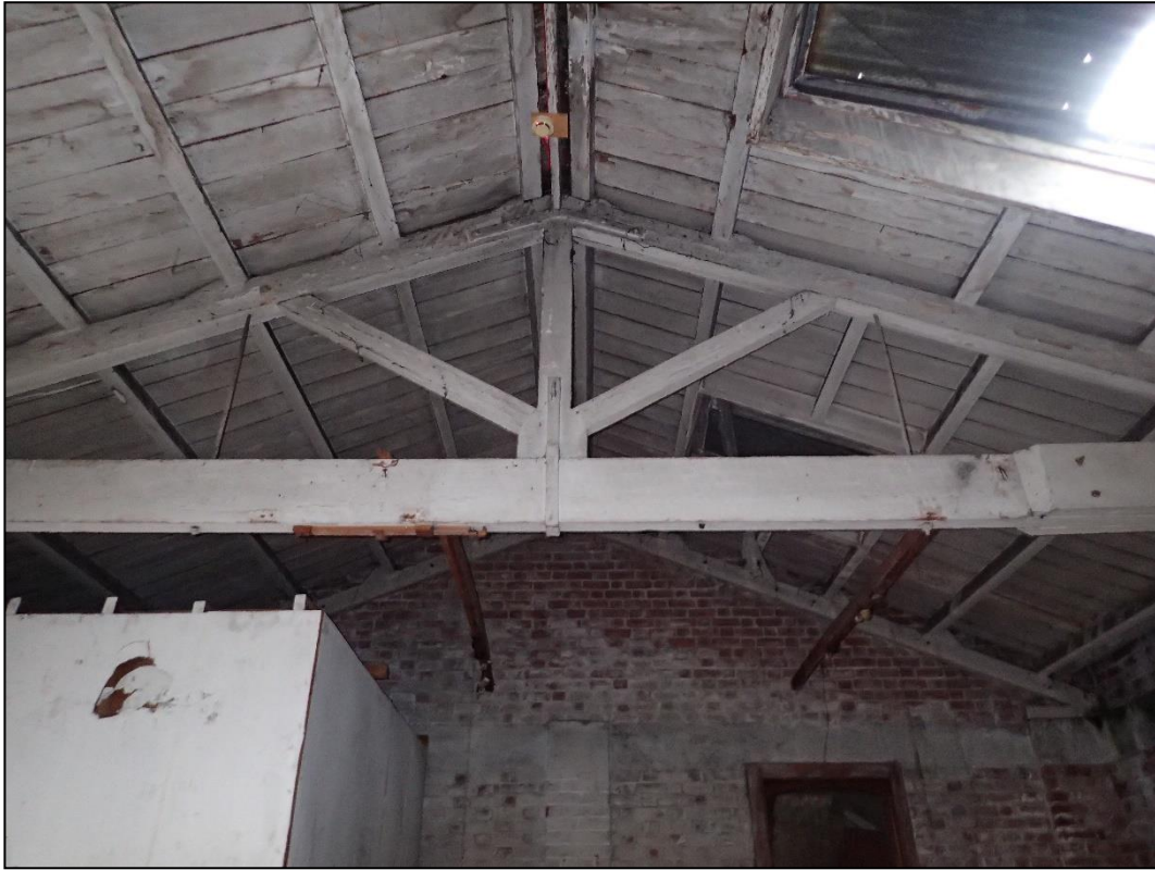
Figure 6-162. The king post truss, purlins and sarking visible in Room 33.
