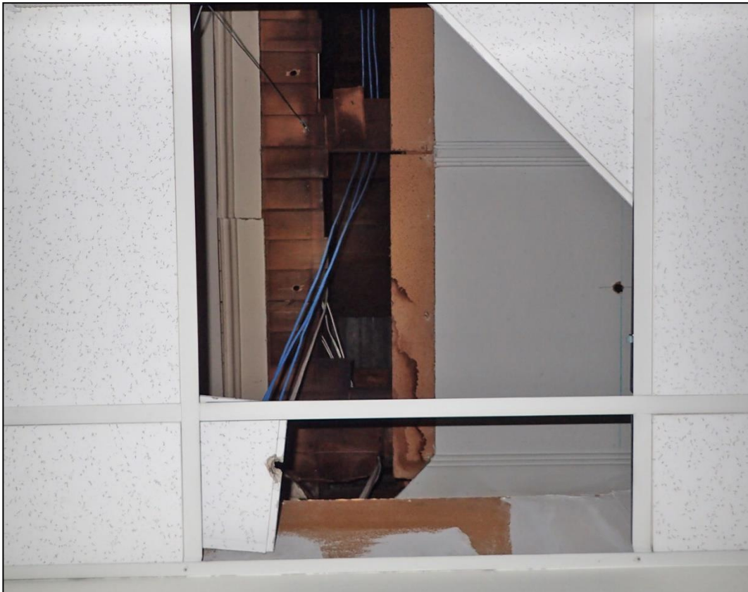
Figure 6-200. Dropped ceiling, earlier softboard ceiling and tongue and groove ceiling in Room 13.
