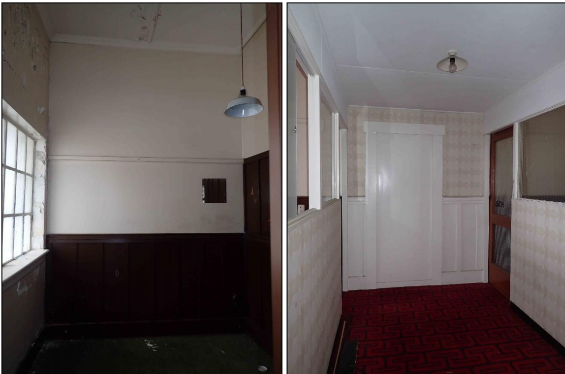
Figure 6-278. Left: Timber wainscoting, dado and picture rail in Room 14. Right: blocked doorway in the east wall of Room 11.
