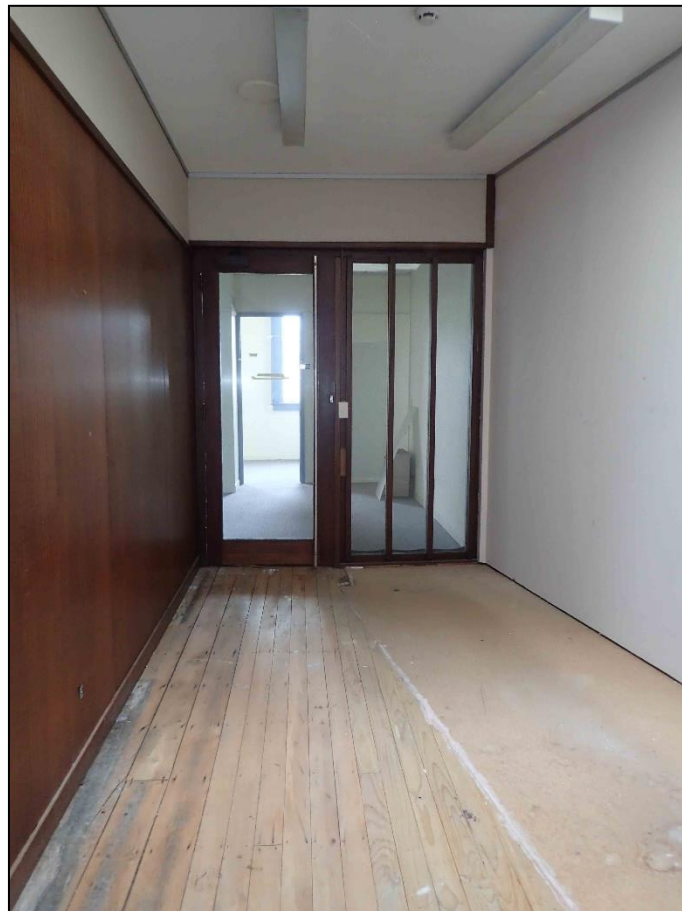
Figure 6-219. Room 24 of the NZIC Building, looking south. Note the scar from the stairwell on the floor.
