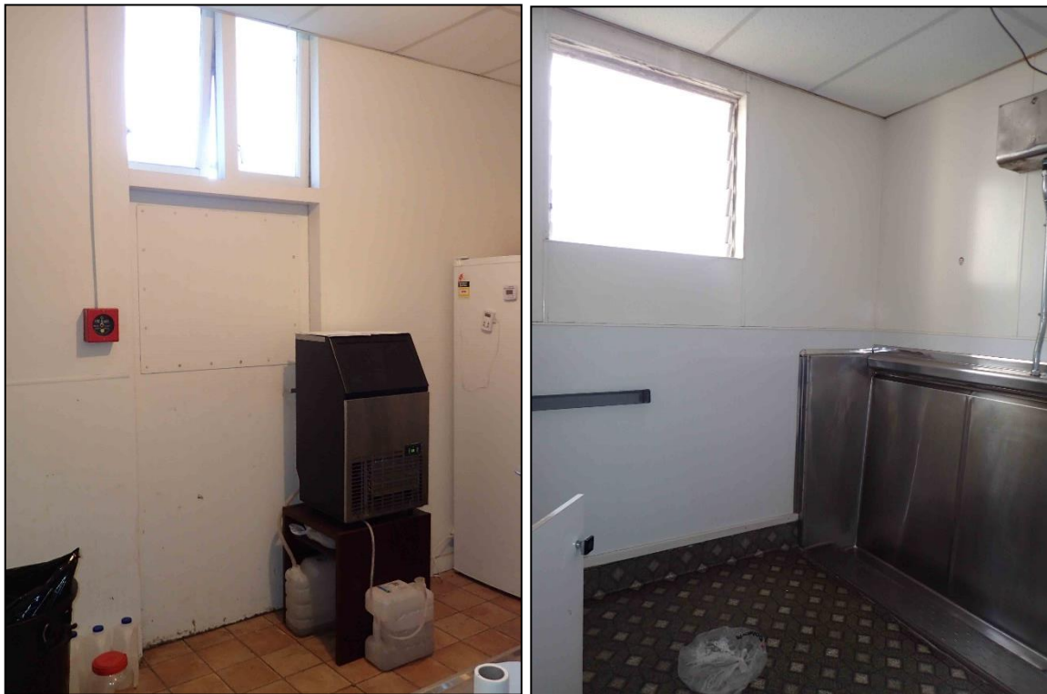
Figure 6-357. Awning transom lights (left) and louvre window (right).
