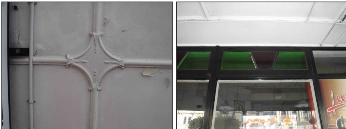
Figure 6-241. Left: fibrous plaster verandah ceiling. Right: stained glass panels on Tay Street shopfront.
