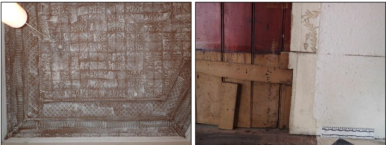
Figure 6-359. Left: pressed tin ceiling in SuziQ's (Room 12). Right: beaded tongue and groove lining and flocked wallpaper in Room 3.
