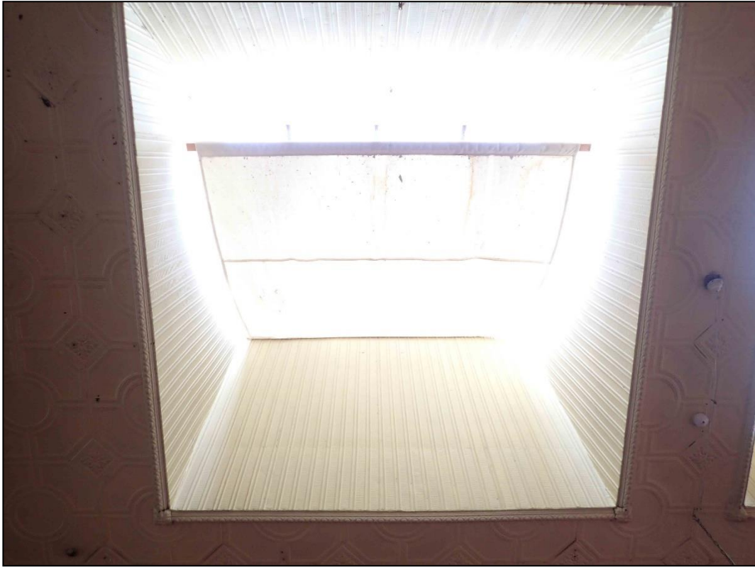
Figure 6-376. Skylight lined with pressed tin in ceiling of 48 Tay Street.
