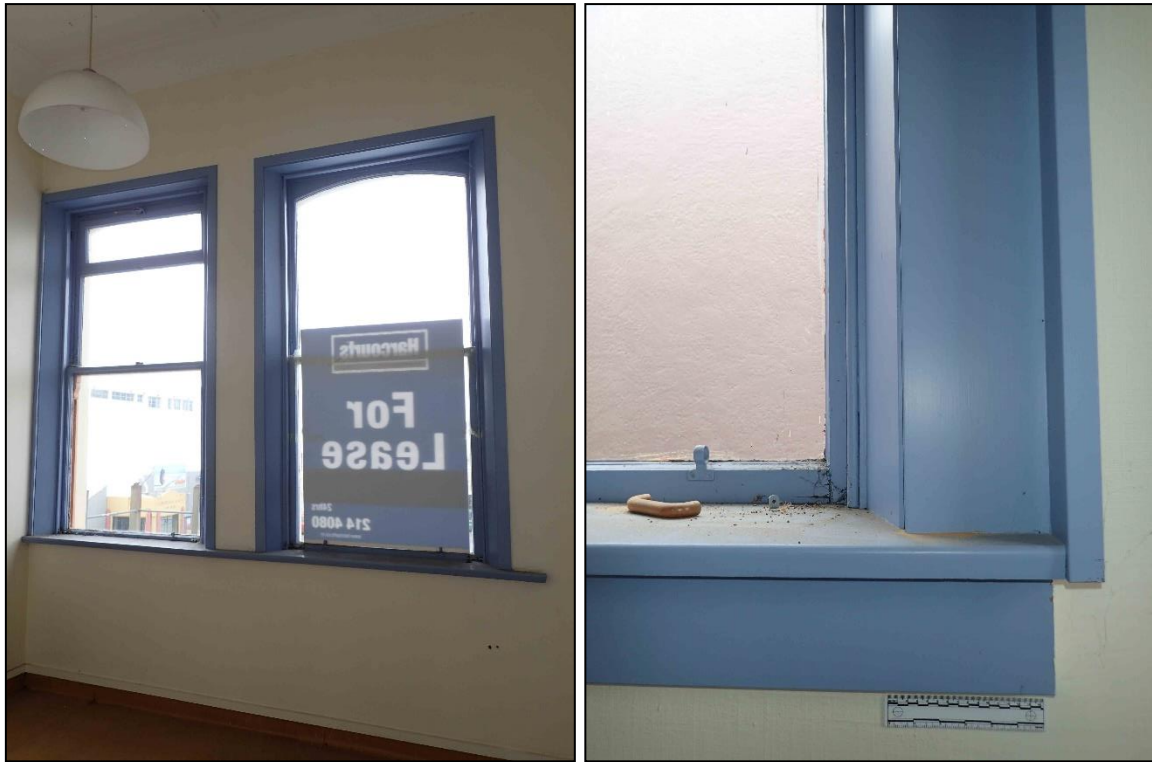
Figure 6-212. Examples of sash windows in the NZIC Building (left) and detail of architraves (right).
