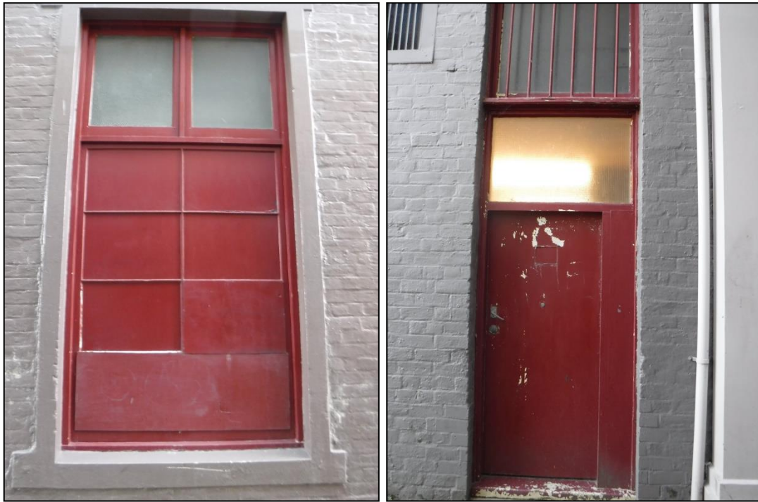
Figure 6-187. Left: The converted loading bay door, Right: modern door in older fenestration.
