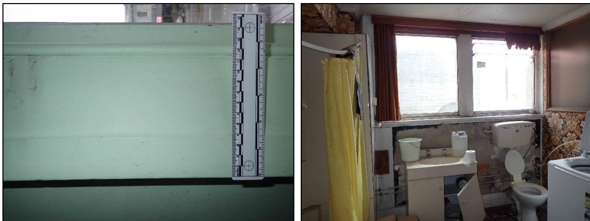
Figure 6-382. Left: detail of architrave on window in Room 9. Right: fixed windows with louvre panes in Room 7.
