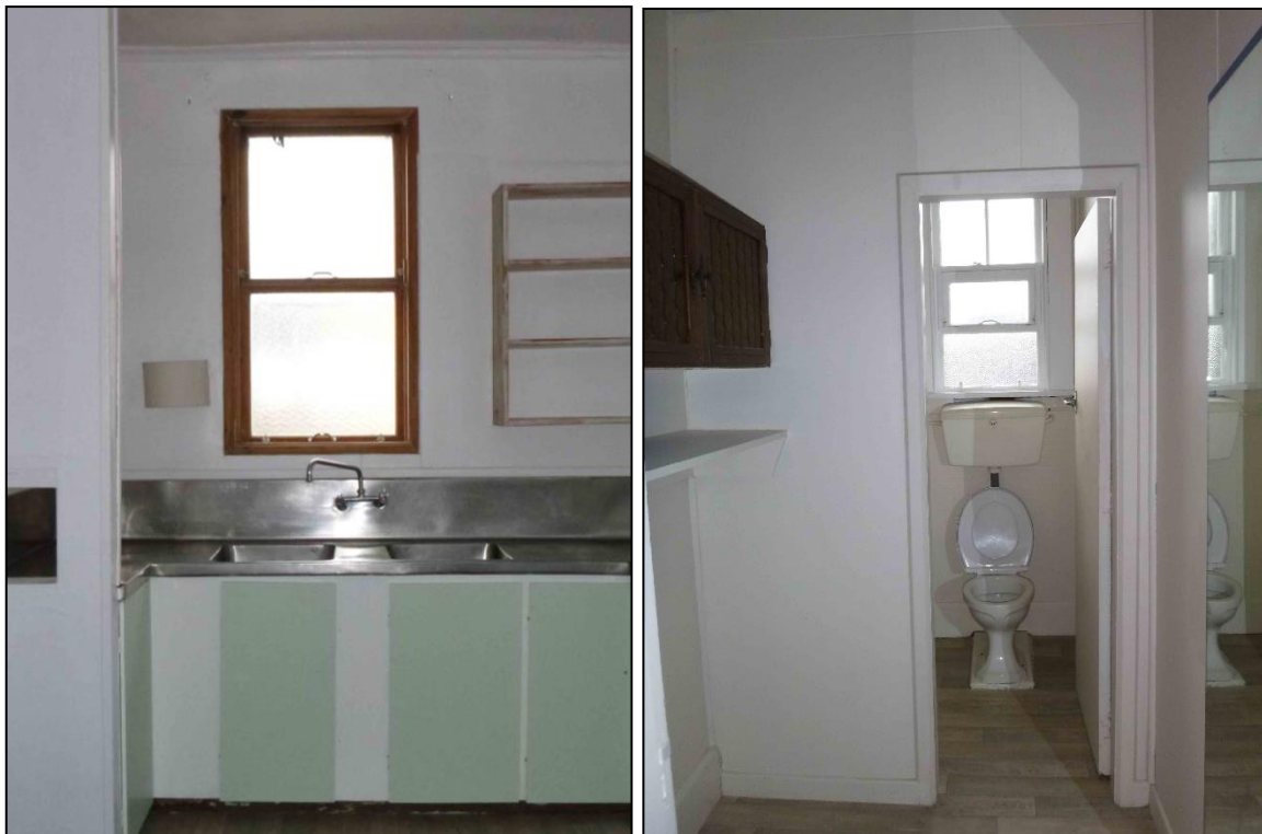
Figure 6-430. Sash window in north wall of Room 13 (left), and altered sash window in north wall of Room 14 (right).
