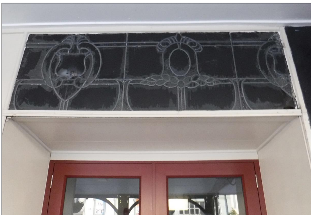
Figure 6-402. Lead light quarter light windows, east end of the south elevation of the Herbert Haynes and Co. Building.
