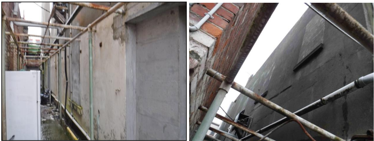
Figure 6-568. Left: the south elevation of the ground floor of Lumsden's Building. Note the filled in windows and doorway. Right: the first floor of the south elevation, looking northwest. Note the line that appears to define the 1876 first floor addition.
