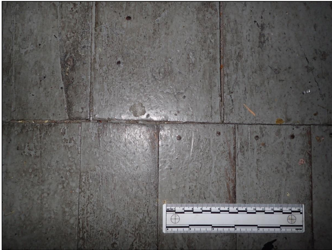
Figure 6-581. Detail of the change in floorboard size from Room 10 (top) to Room 12.
