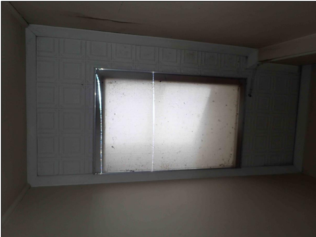
Figure 6-464. Pressed tin ceiling and skylight in Room 3 of Kingsland's Shop.
