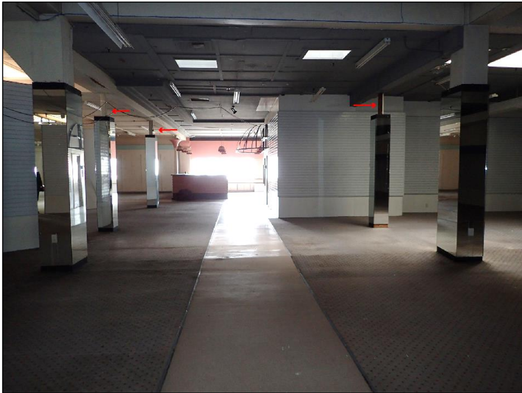
Figure 6-411. Looking south in Room 2 of the Herbert Haynes and Co. Building. The red arrows indicate cast iron ceiling posts.
