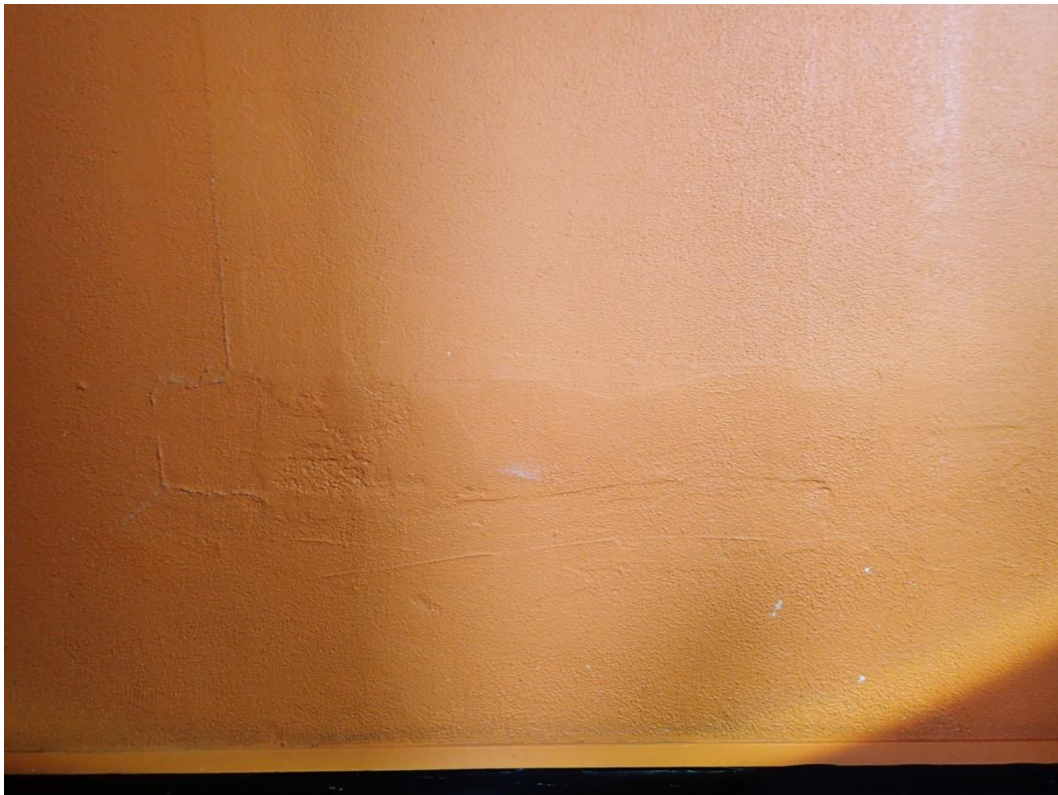
Figure 6-574. Scarring where the window sill has been removed from the original exterior of the east elevation.
