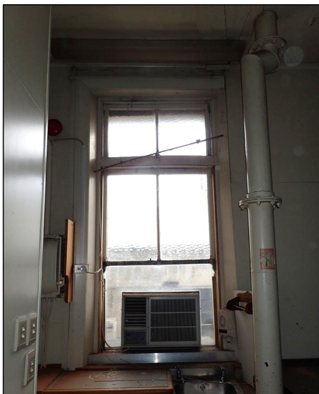
Figure 6-413. This modified sash window in the west wall of Room 2 appears to be an original feature.
