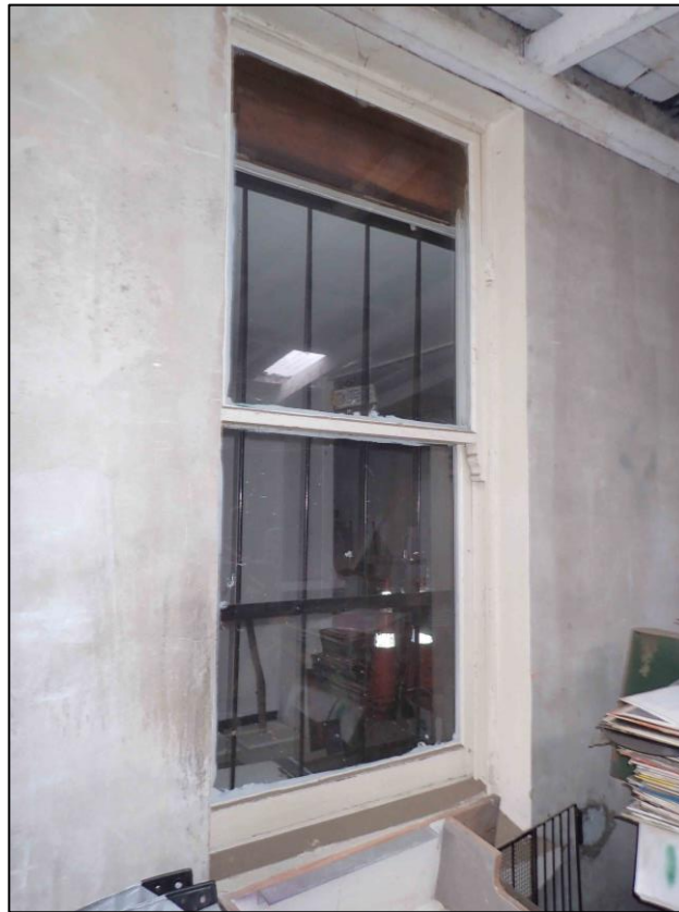
Figure 6-484. Original timber sash window with lugs in ground floor north elevation.
