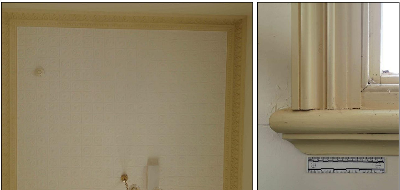
Figure 6-544. Left: the pressed timber ceiling of the second-floor landing. Right: the original stool and apron with a modern architrave.
