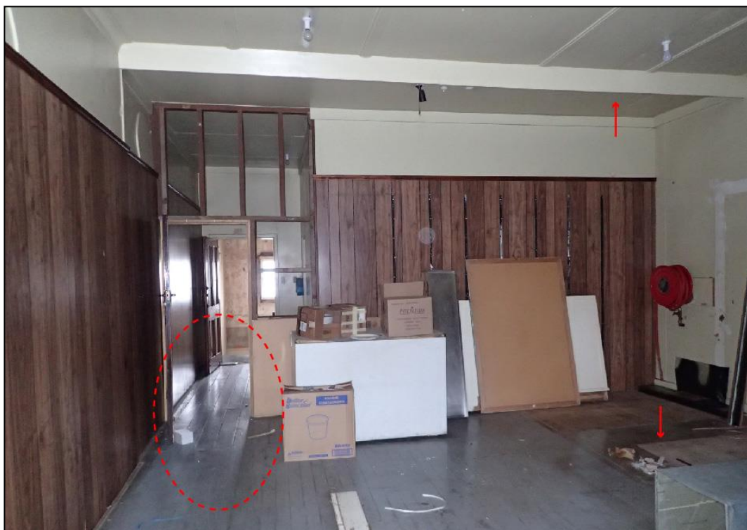
Figure 6-580. Looking east in Room 12 toward Room 10 with the change in floorboards circled in red. The arrows indicate scarring in areas where walls have been removed.
