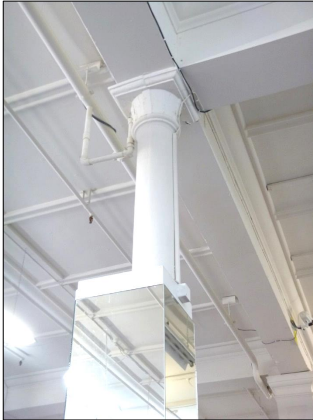
Figure 6-409. Example of a cast iron ceiling post in Room 1.
