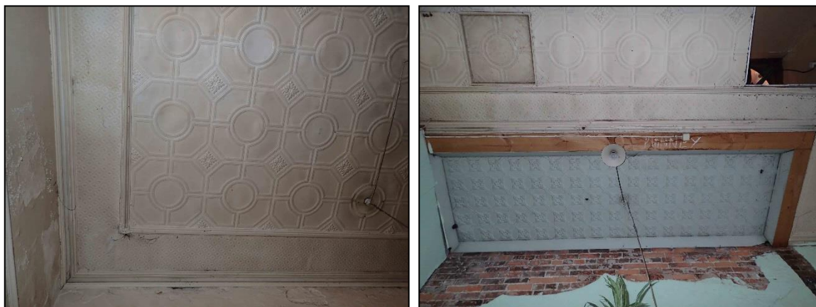
Figure 6-387. Pressed tin ceiling and moulded cornice in Room 9, with old stairwell ceiling (right).
