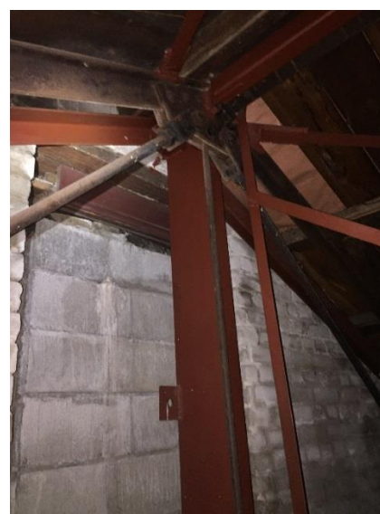
Figure 24 – West Gable front element strengthening girt has no effect on outwards movement as no fixing to wall and only at one location.
