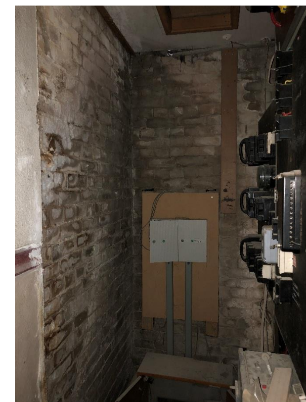
Figure 20 – Ground Floor North West corner evidence of efflorescence to the brickwork internal leaf.
