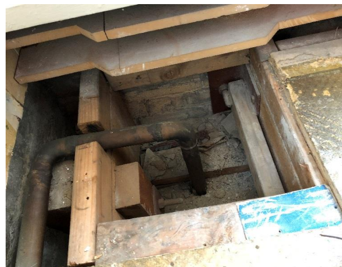
Figure 22 – North and East Elevation ties into floor diaphragm at first floor. Façade tie local to trimming joist only, minimal transfer path. East elevation fixings every second joist
