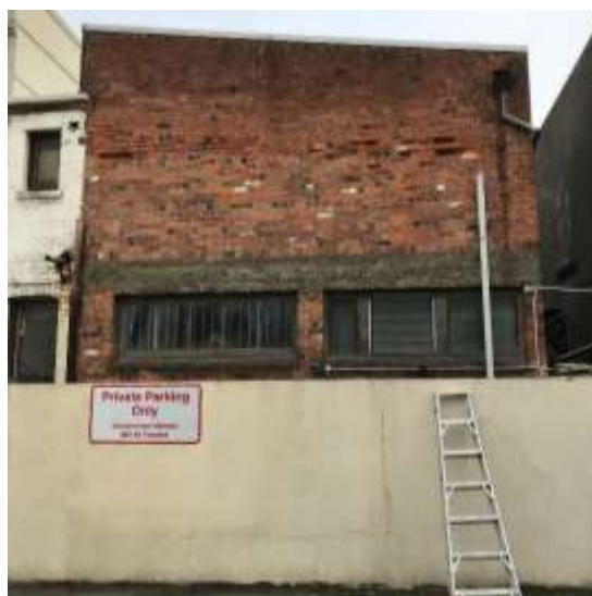
Photo 1: Rear of building showing second floor elevated roof section.
