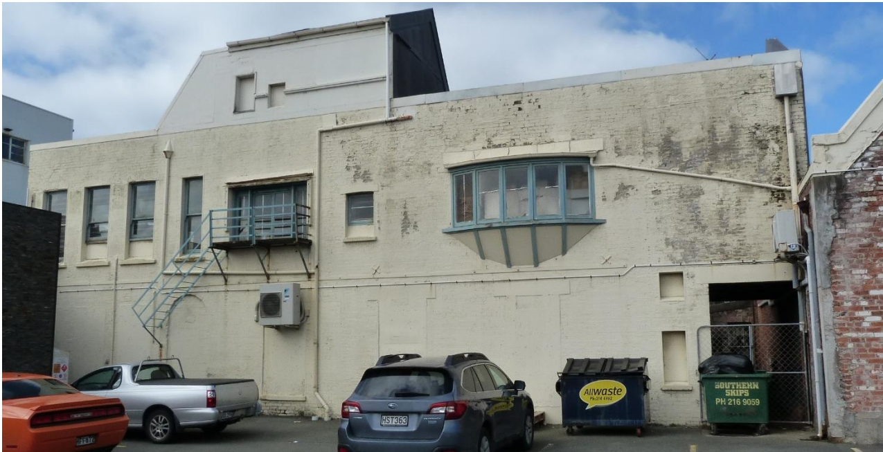
Photo 1: Rear of building showing elevated roof section & some tying of timber mid floor to brick walls visible (steel strap & fixings).
