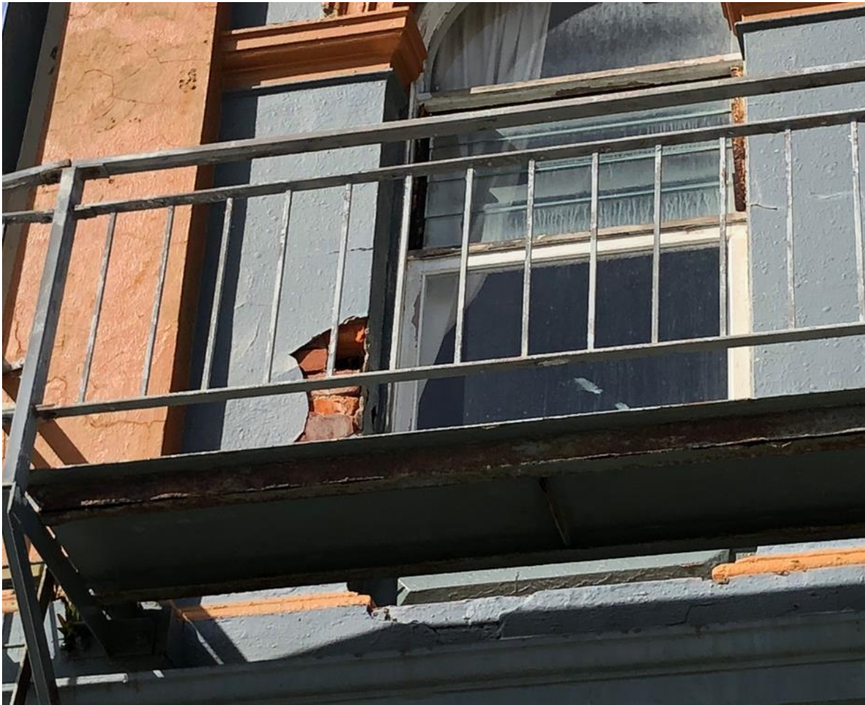
Fig 6.0; see the weathered bricks adjacent to the upper windows, there is no strength left in these bricks, the crumbling of plasters are significant with bricks being dislodged with weathering and damage which precludes these walls from any structural maintenance or refitting of new bricks as the bricks themselves have lost their inherent strength and no bond at all is left between any courses adjacent.
