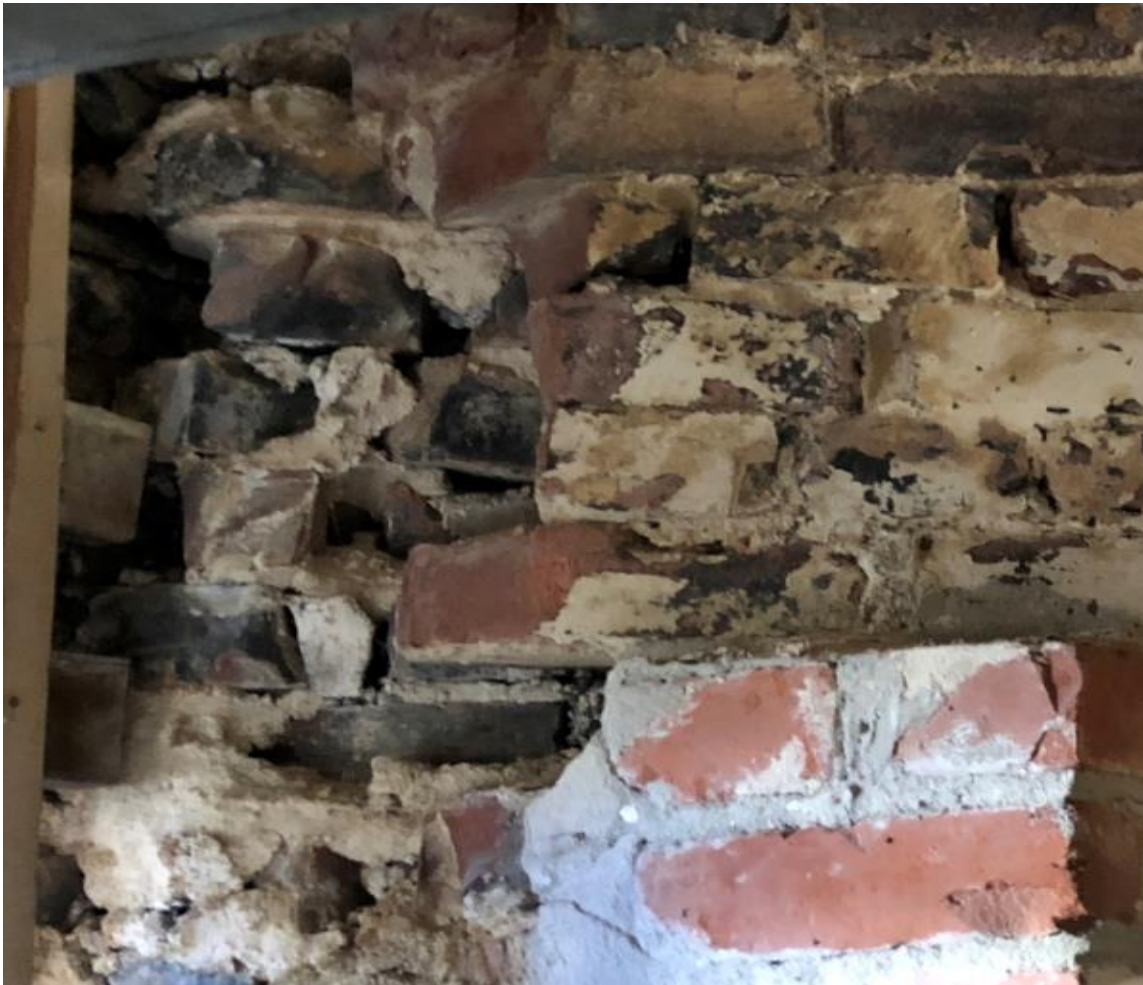
F13; Rubble of bricks are shown with poor cemented interlacing to the front bricks, such situations in this building is common.
