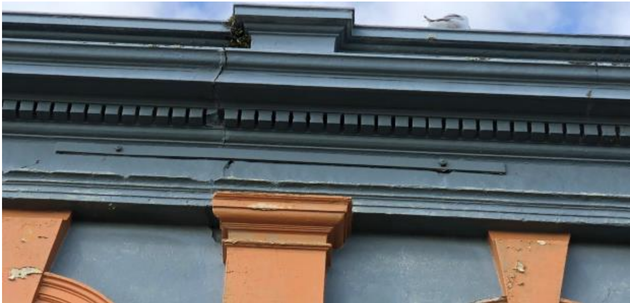
Fig 11.0; See the vertical shear cracks where the steel bar has been placed to limit future cracking, but unfortunately this will do little to stop cracking continue to plague this whole parapet.
