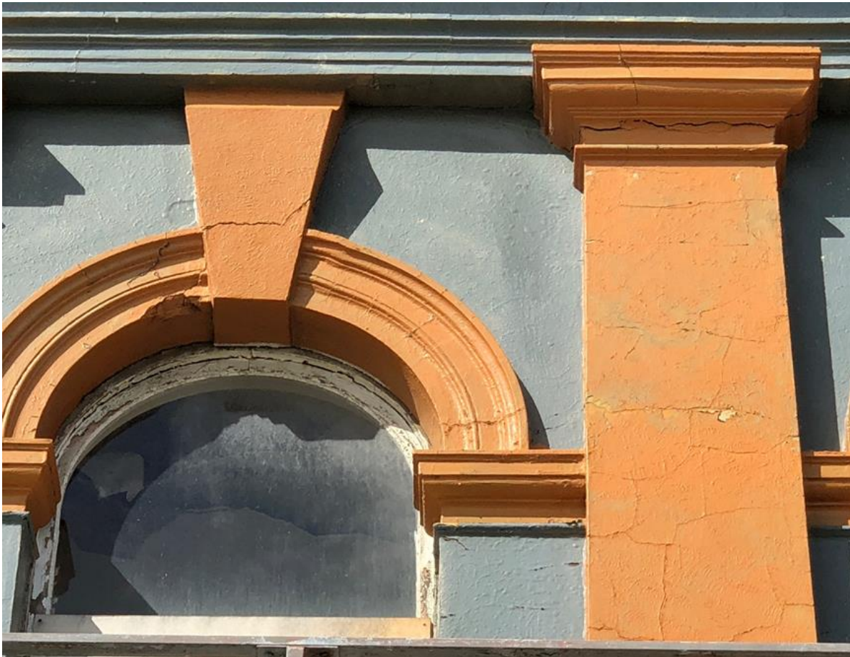
Fig 8; The cracking around the decorative corbels is not just through the plaster but such cracks go right through into the bricks placement which was poorly built from day one, the numerous cracking means large sections of these plastering features are able to come a drift with continual weathering over time and it is just typical of this whole front facade.
