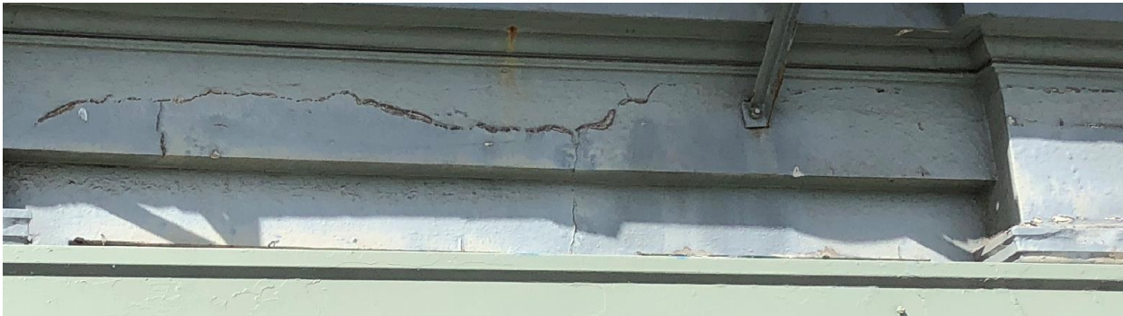
F15; Note the horizontal cracking through the lintel
