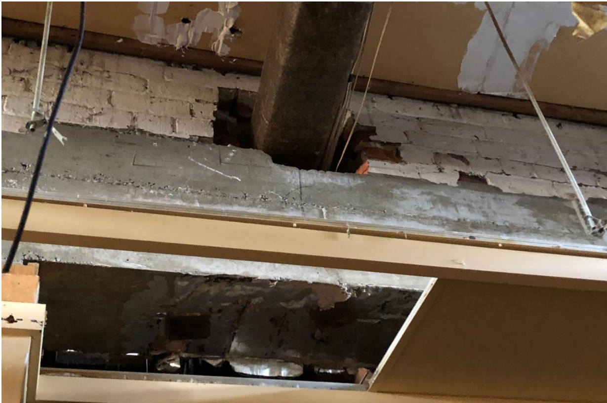
F 1.0 Historic entries for newer ducts have caused major structural damage which has tried to be fix with insut concrete but the bricks at the interface are crumbling.
