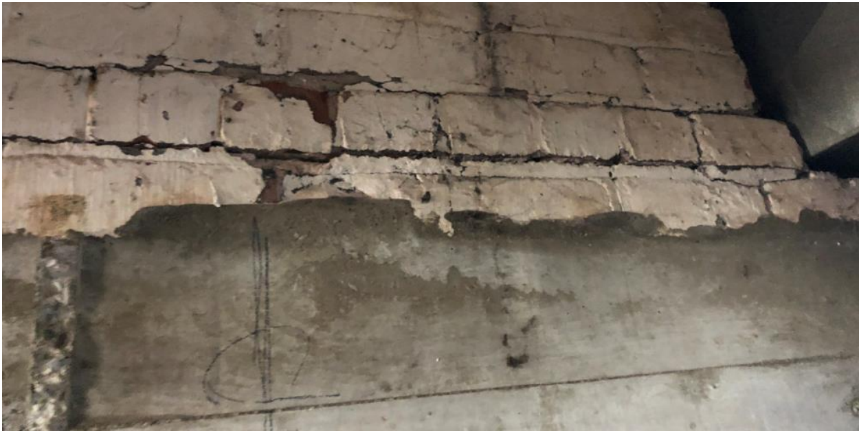
F16; There exists horizontal cracking through the brick courses which results from poor failed mortar and no doubt historical EQ loads exceeding the strength of the in place brick shear walls, or these courses could well have dropped at the similar time the concrete section of the new base lintel was poured. These part concrete lintels as placed in sections through the lower floor will contribute to significant weakening of the whole building.
