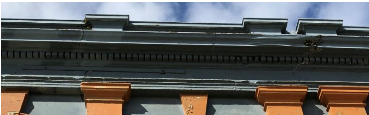
F7.0; There are numerous complete shear cracks between the upper lintels / parapets to make them ready to topple off and go through the ground veranda to the pavement, wind could well move such large parapets and hence this supports the argument that the building is now dangerous.
