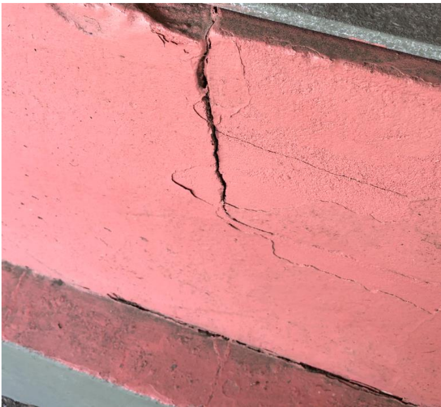
F 2.0 Major cracks in unrienforced foundation beams make it difficult to consider any strengthening solution as load paths to the ground have been compromised.
