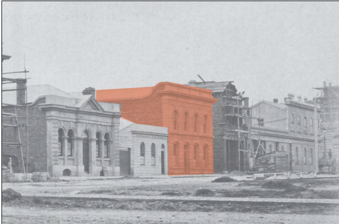
Figure 4-24. Detail from a late 1878 photograph showing building on 12-14 Esk Street highlighted in red (Southland Museum and Art Gallery, 1878).
