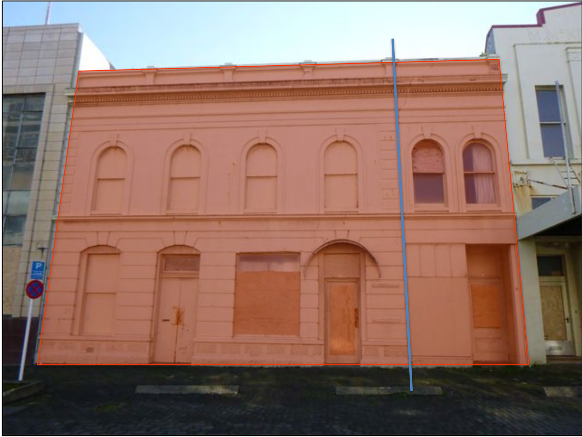
Figure 4-26 Current view of the former Southern Cross Building (12-16 Esk Street). Note the boundary as indicated by the blue line between the two buildings on Lots DE (left) and F (right).
