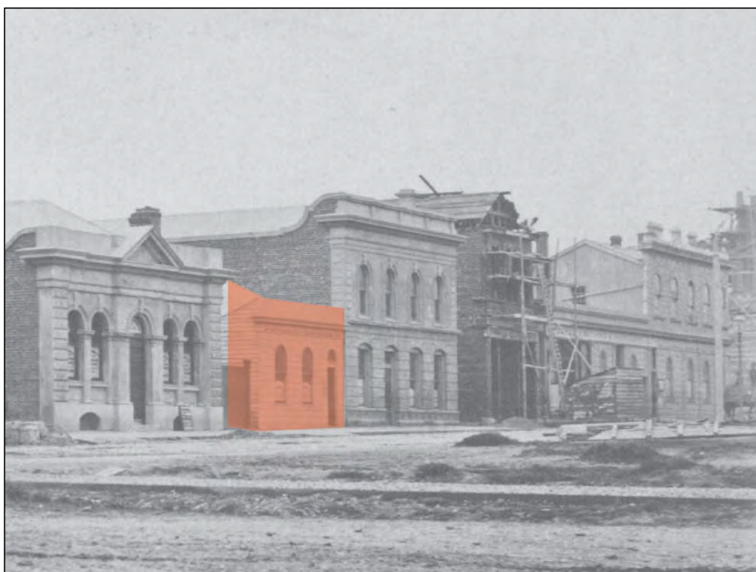
Figure 4-21. Detail from late 1878 showing building at 10 Esk Street highlighted in red (Southland Museum and Art Gallery, 1878).
