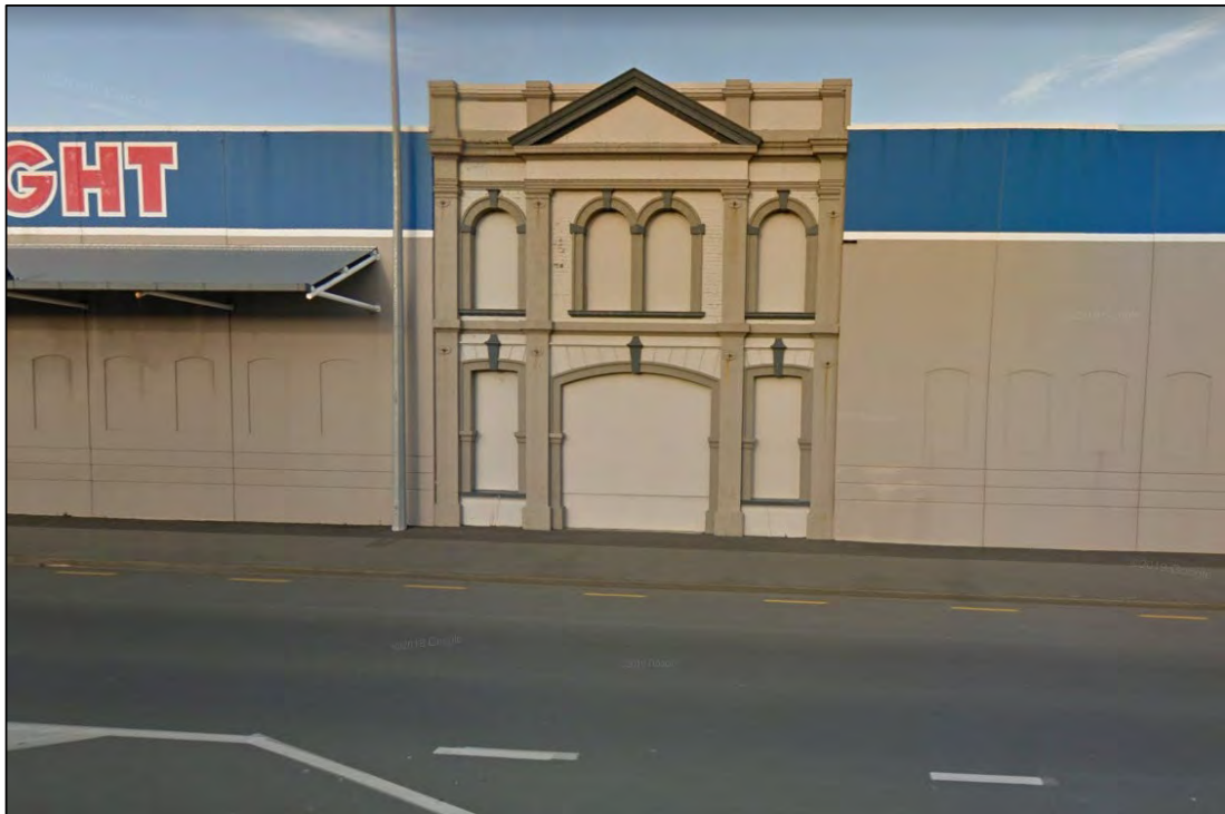
Figure 7-3. An infamous example of façade retention in Invercargill within the Spotlight building at 33 Leven Street.
