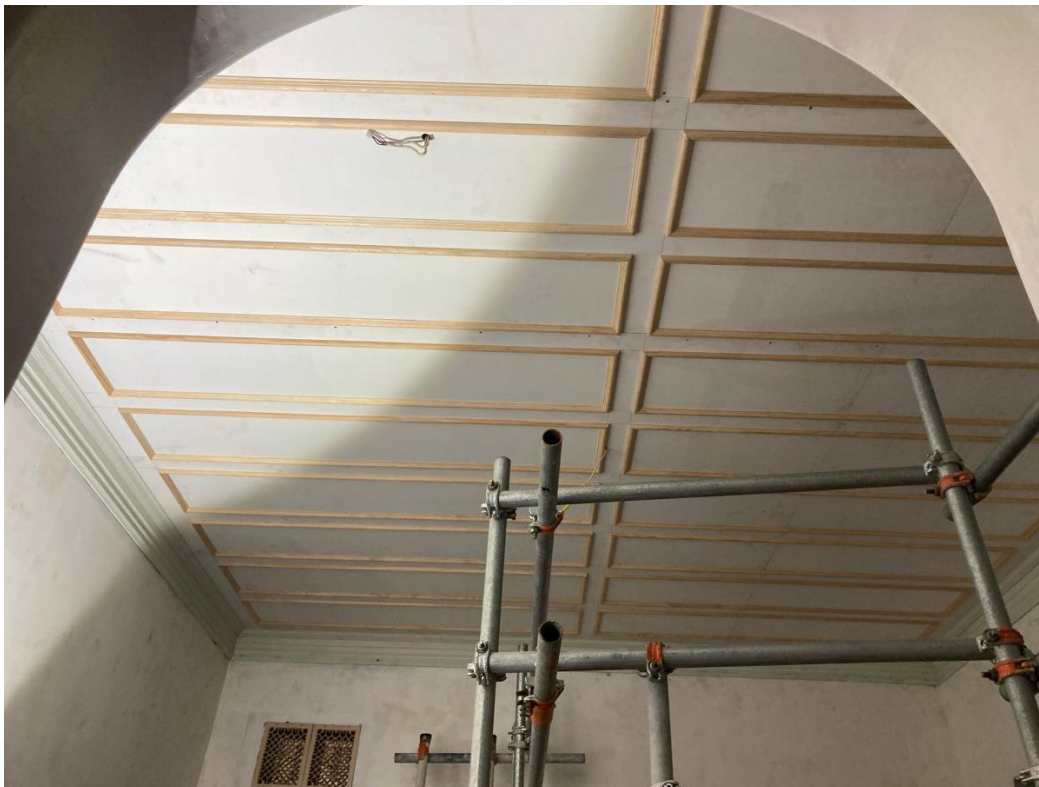
Figure 2 – First storey stairwell ceiling during refurbishment
