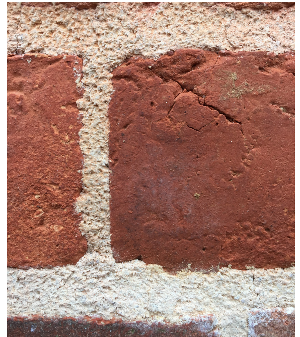
An example of good, flush pointing using a hot-mix lime mortar.
