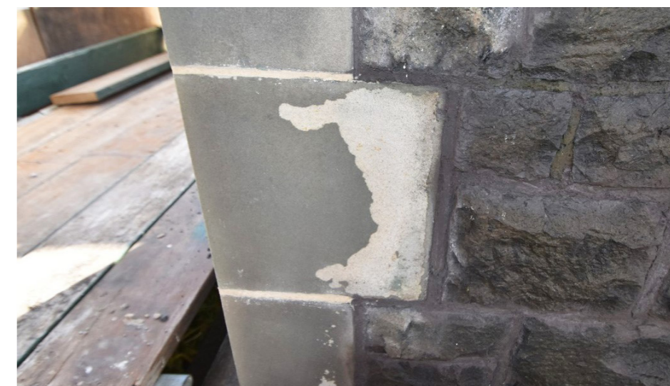
A previously applied sealant has attracted pollution on the quoin, forming a dark skin that is no longer capable of being cleaned
