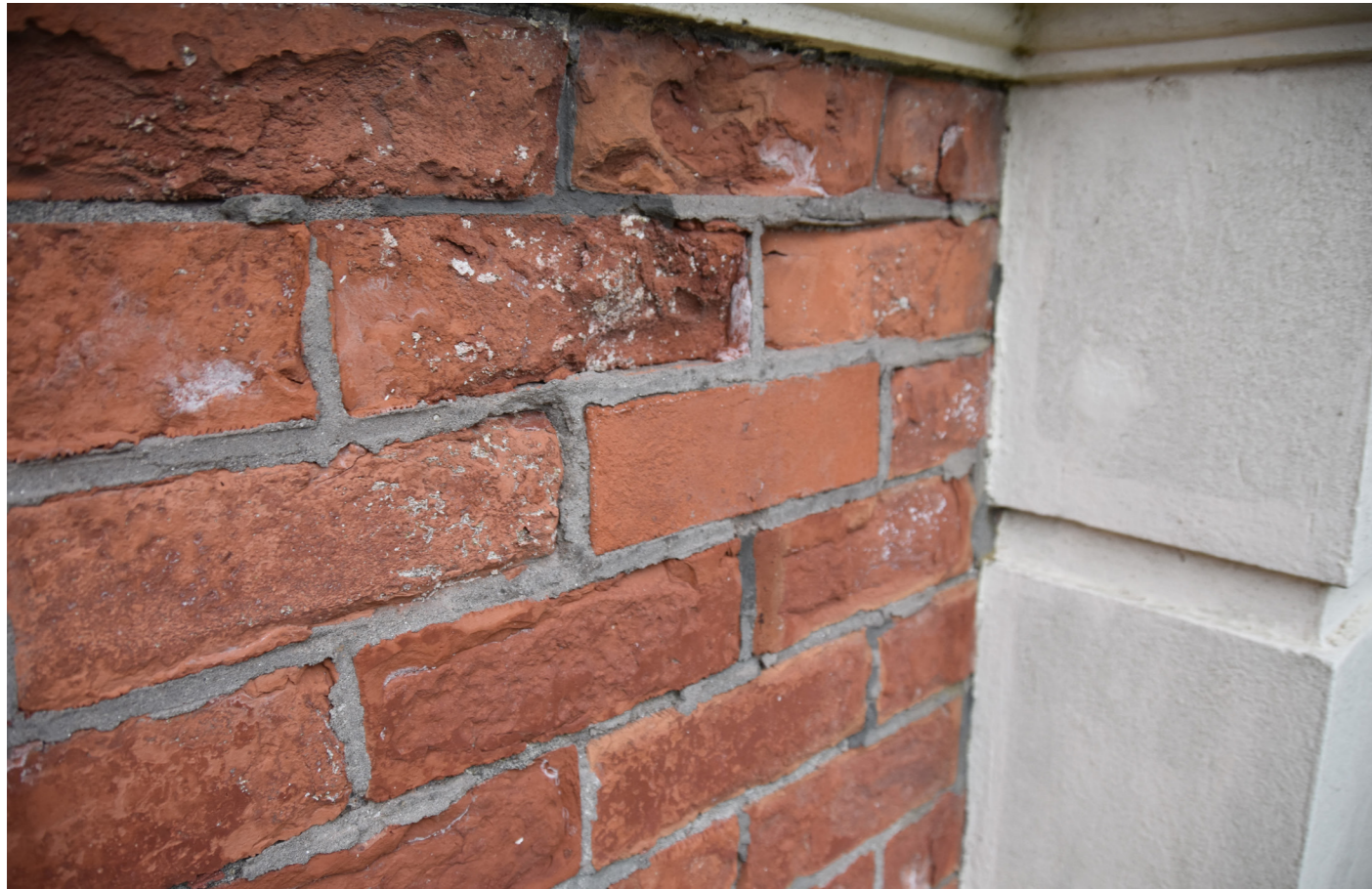
Above: Bad cement pointing and associated brick decay and the presence of white salts/efflorescence.
