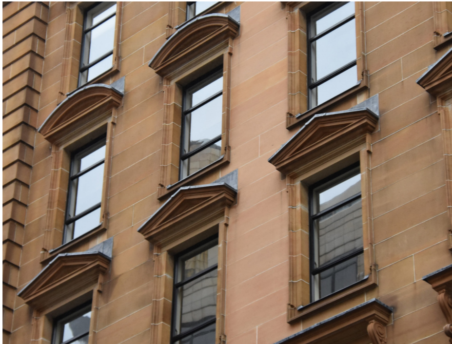
New lead flashings applied to tops of window pediments and ledges
