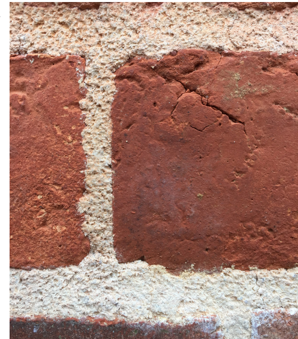
An example of good, flush pointing using a hot-mix lime mortar.
