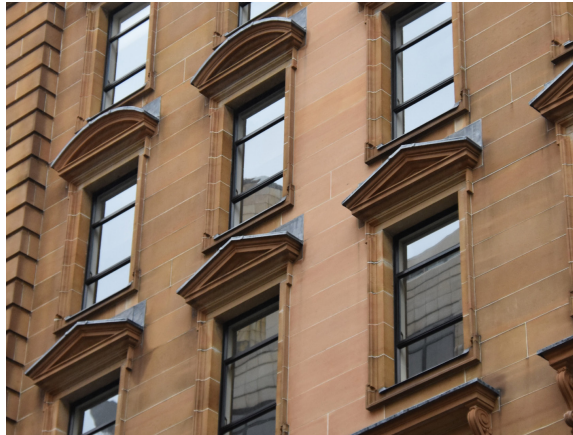
New lead flashings applied to tops of window pediments and ledges
