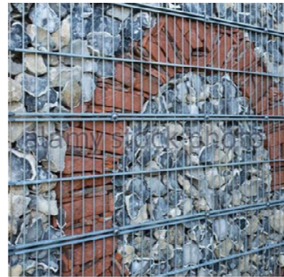
Feature rubble filled gabion wall*
