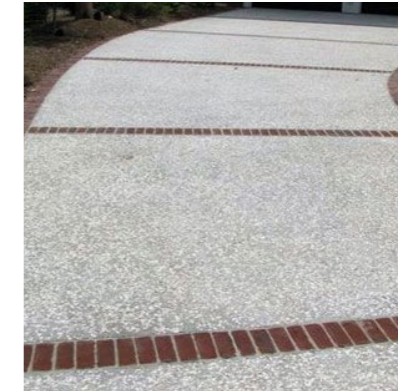
Crushed oyster shell mixed with concrete
