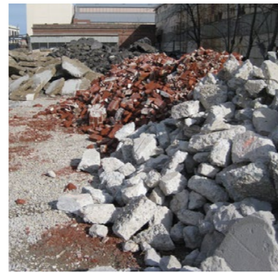
Club Hotel rubble to be re-used on site
