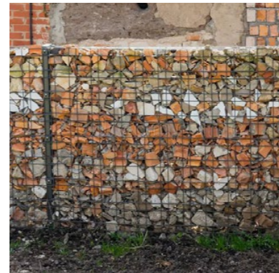
Rubble filled gabion wall*
