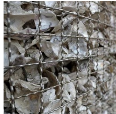
Oyster Shell filled Gabion Wall*
