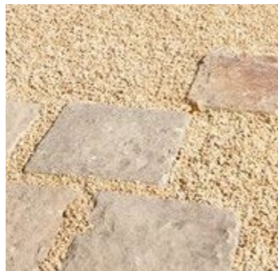
Crushed material or hoggin between larger found materials.
