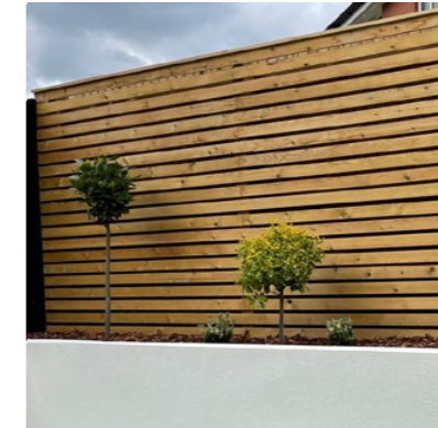
Batten timber fence
