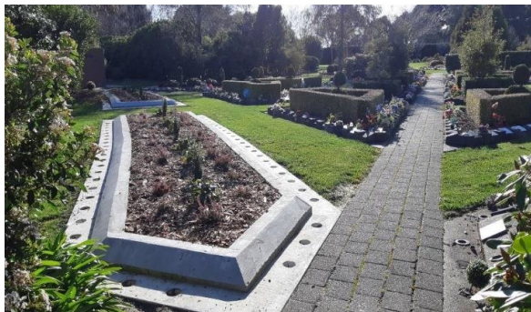
Figure 6: Two new beams in the Garden of Rest
