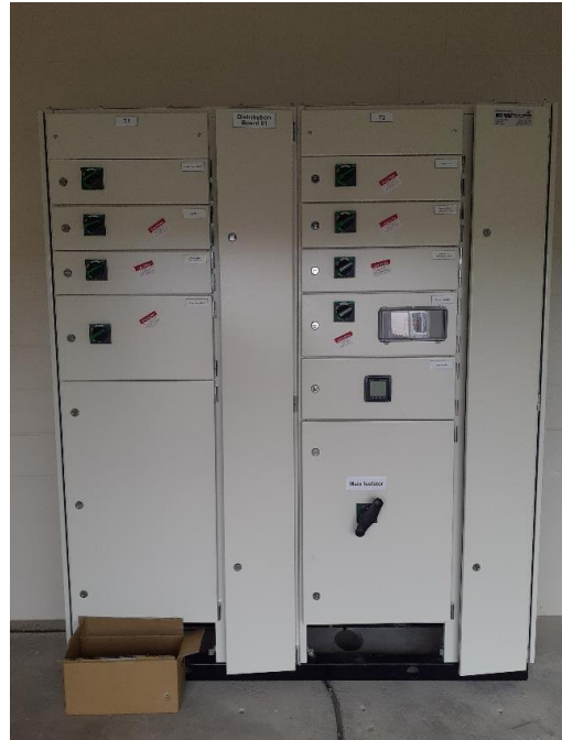
New primary switchboard for equipment mains isolation
