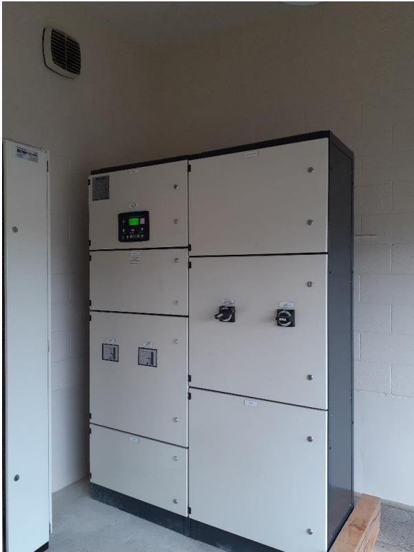
New primary switchboard for equipment mains isolation
