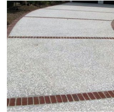
Crushed oyster shell mixed with concrete
