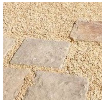
Crushed material or hoggin between larger found materials.
