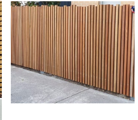
Timber feature fence
