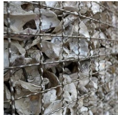
Oyster Shell filled Gabion Wall*
