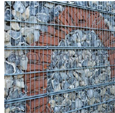
Feature rubble filled gabion wall*
