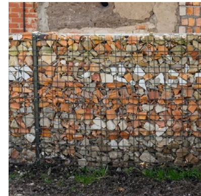
Rubble filled gabion wall*
