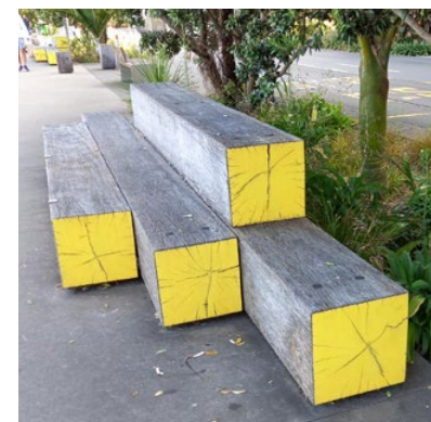
Chunky steps and seating made from wharf materials
