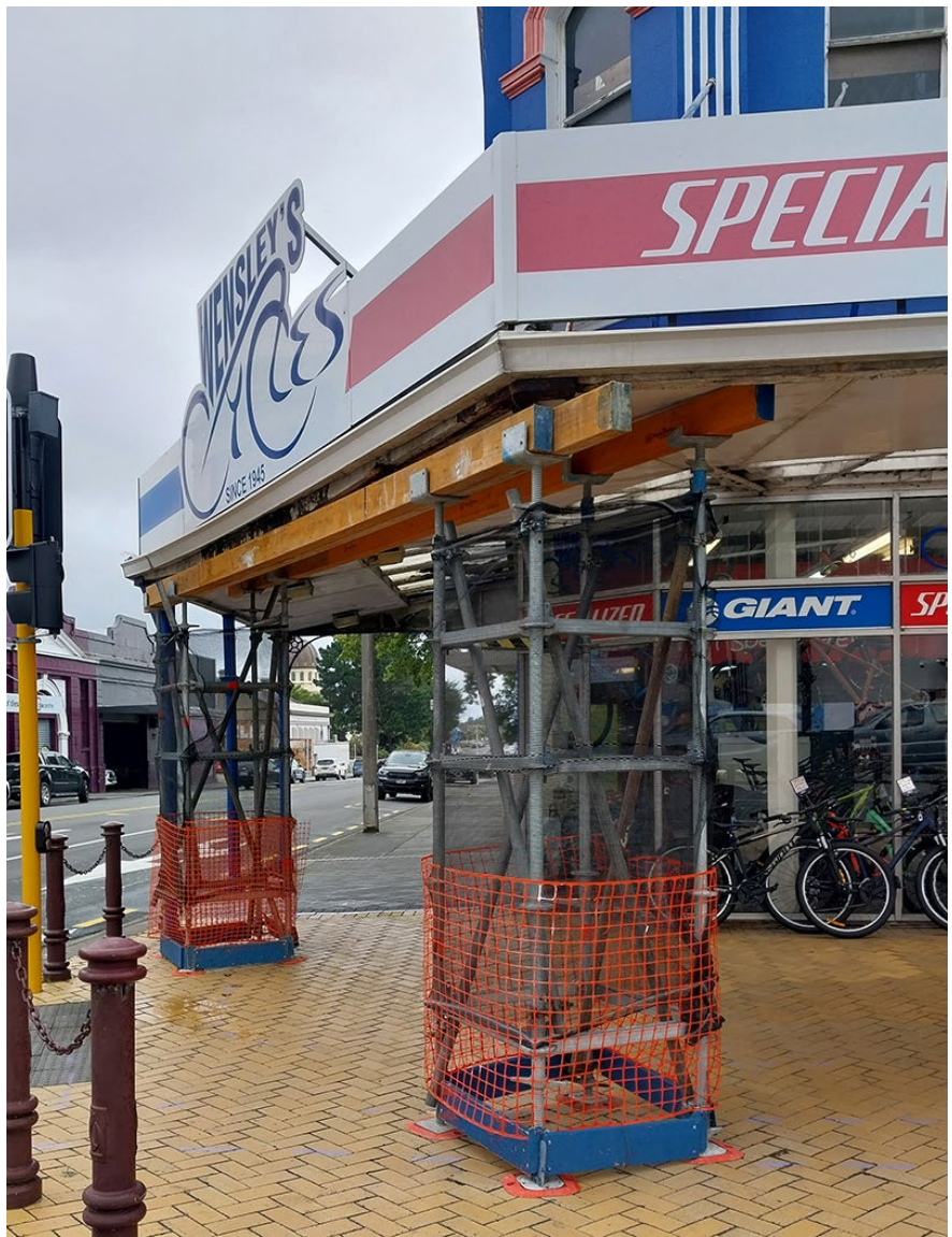
The verandah has been temporarily propped up until repairs can begin.
