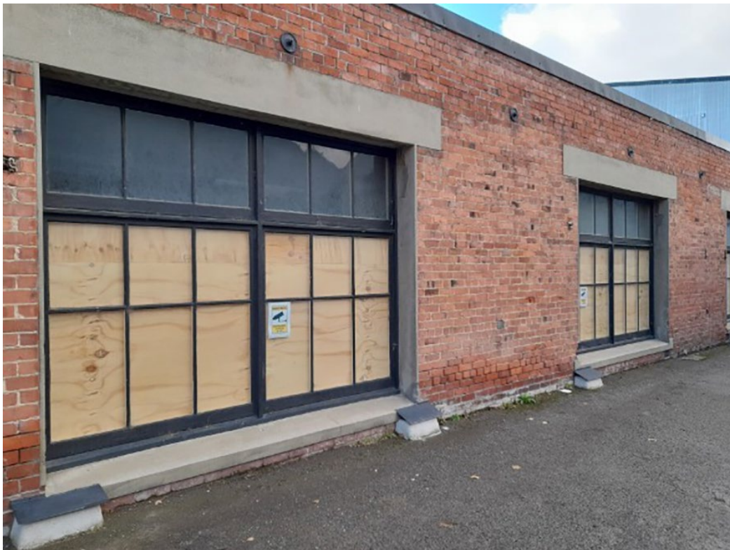
Eastern windows along alley – plywood sheathing has been put against them to protect against vandalism. This is not an ideal heritage outcome.
