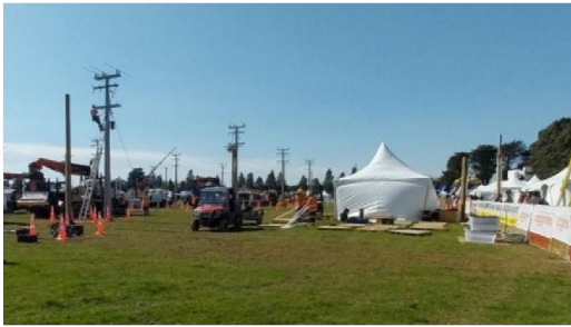
Fig 3: Power poles installed as part of the Annual Connexis event.
