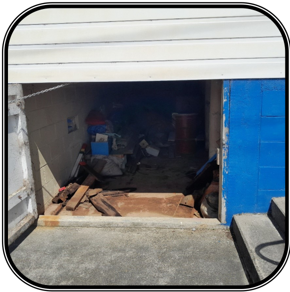
Access to underfloor area/ storage, No insulation or vapor barrier present
