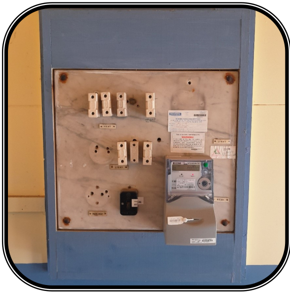
Older style switch board with porcelain fuses
