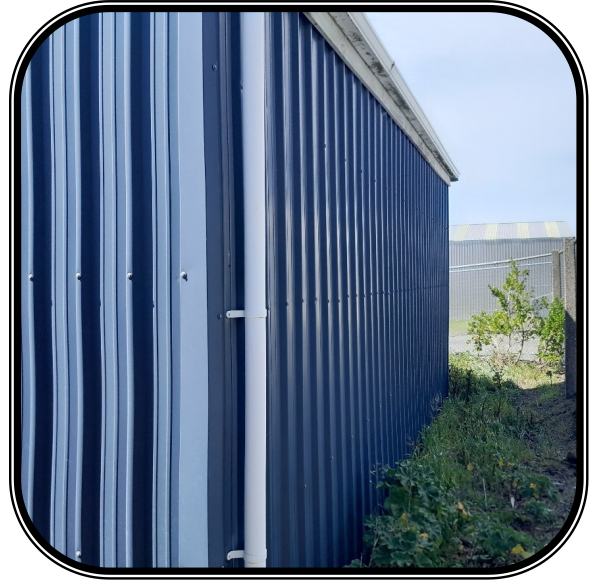
Soil in direct contact with cladding south end of building
