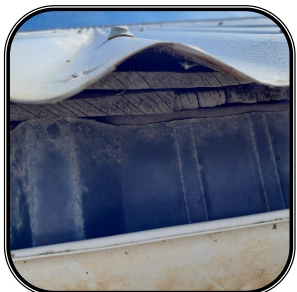
Roof iron installed over original shake tile roof, cladding top seal/ flashing detail incomplete
