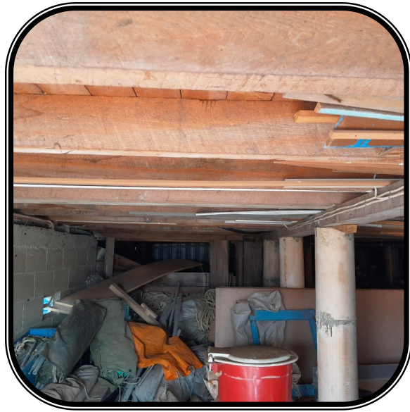
Standard concrete pile and ring foundation construction, timber sub framing
