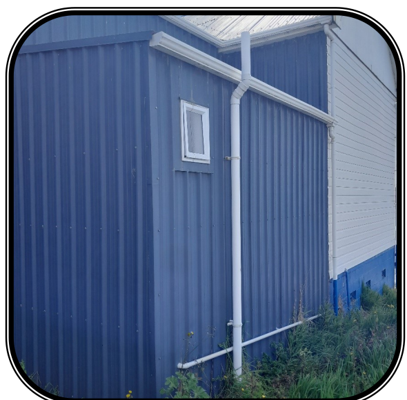
East side cladding change over from colorsteel to pallside
