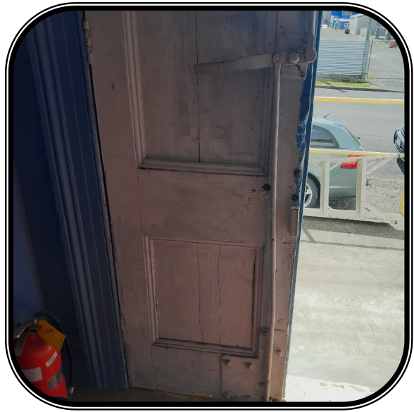
Antiquated hardware/ escape bar, this will be non operation while the exterior slide bolt and padlock are secured
