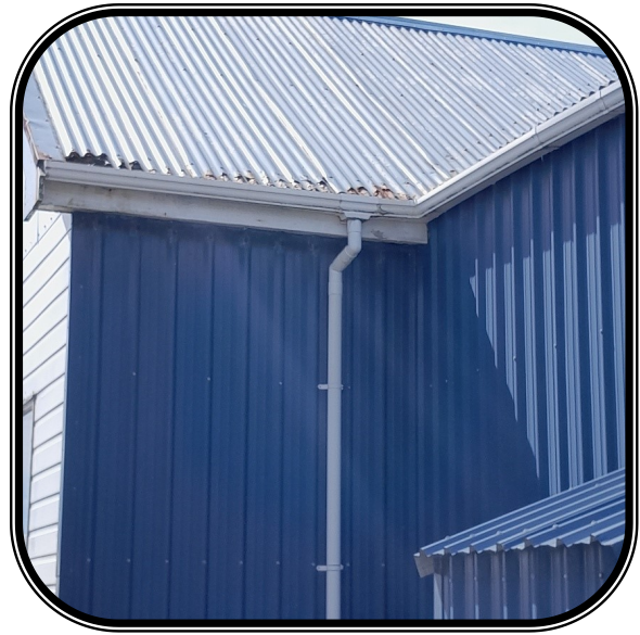
Deteriorating roof cladding
