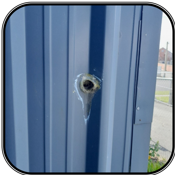
Unsealed penetrations through cladding, visible in a number of areas around building
