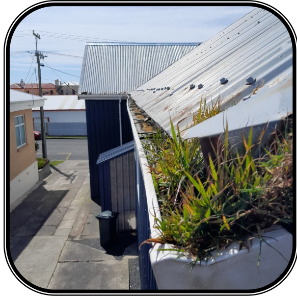
Repairs and clean of gutters required
