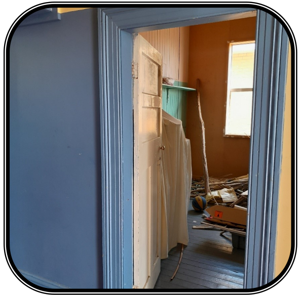
West room utilized for storage, no ventilation, hardboard linings
