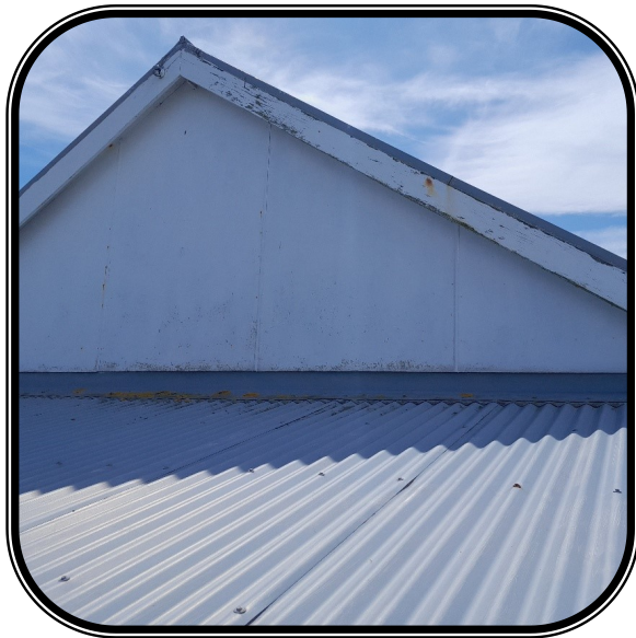
Rear over stage roofing reasonable condition, secured with lead head nail
