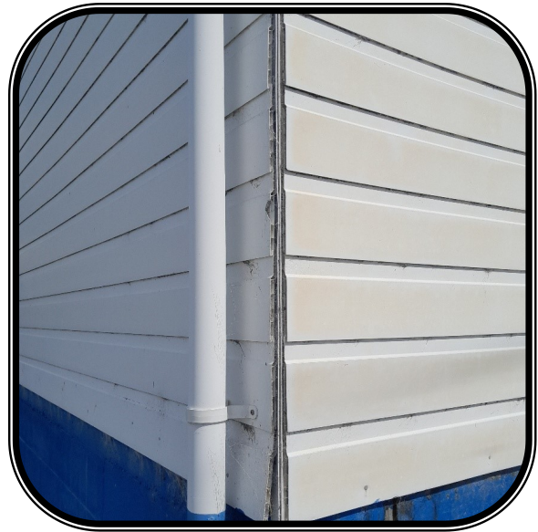
Corner flashing missing from cladding system
