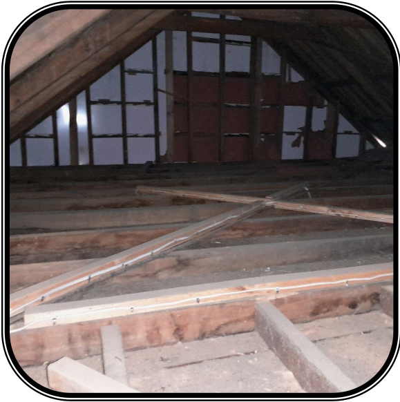
Roof cavity, no insulation present
