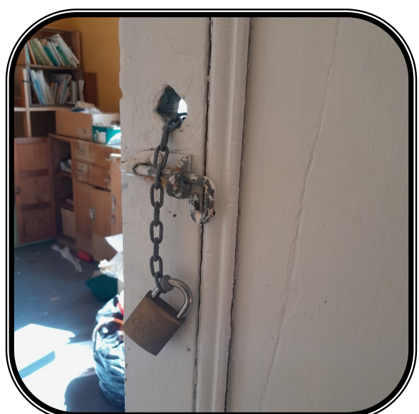
Door hardware non operational, secured with slide bolt and padlock
