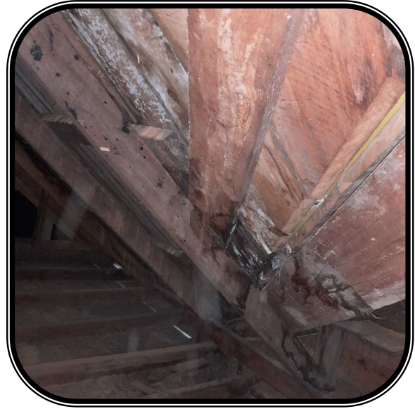
Signs of water damage from roof leaks
