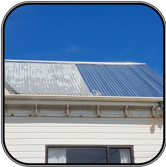
Section of roofing replaced
