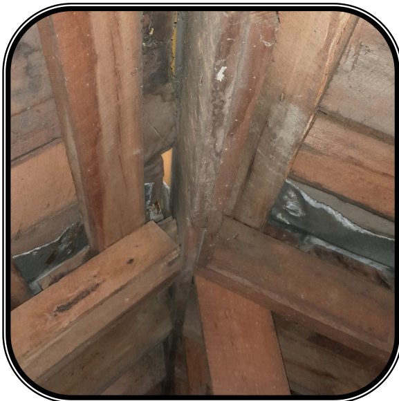
Daylight visible through ridge line and visible deterioration to roof cladding
