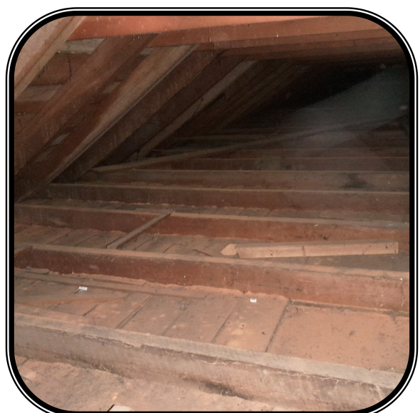
Signs of borer in roof framing/ ceiling linings
