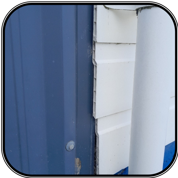
Connection between two cladding systems incomplete, exposed end to pallside cladding
