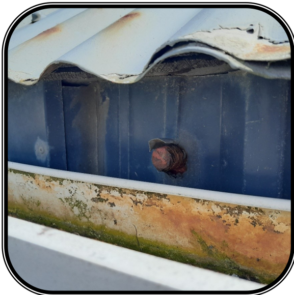
approx. 75mm drop from roofing to spouting, exposed collar tie rods through cladding corroding and unsealed penetration
