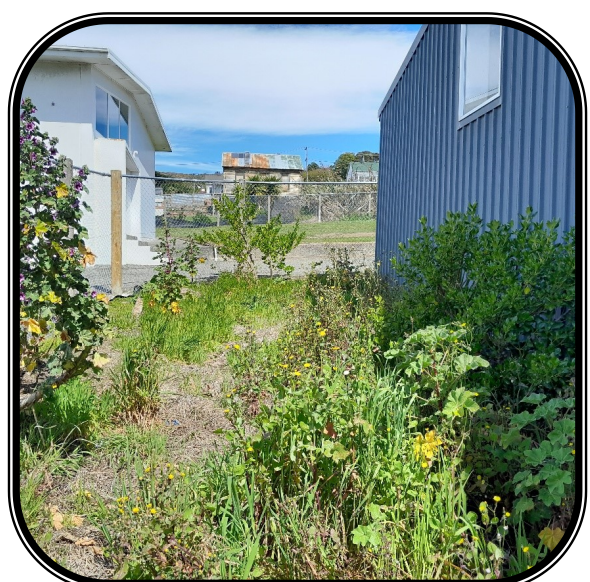
Vegetation in contact with cladding, including soil at rear end of building in direct contact with cladding
