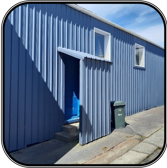
Wast side of building , rear cladding in contact with ground
