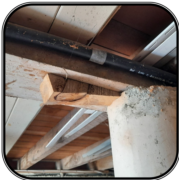
Some settlement noted which has been blocked and wedged in places
