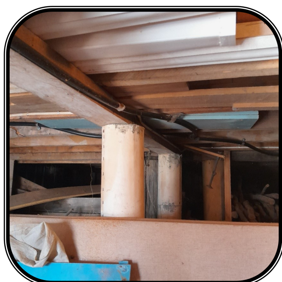
Borer noticed in framing however still structurally sound
