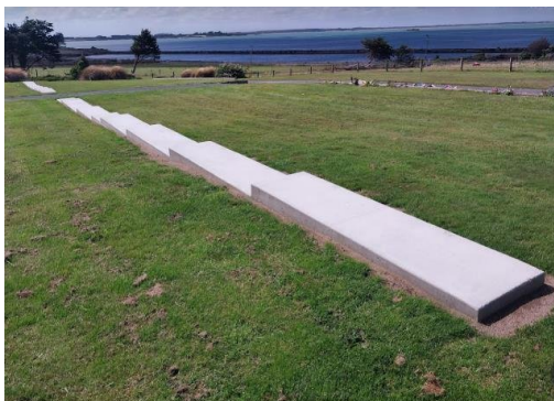
Figure 5: New burial beams at Greenpoint Cemetery.
