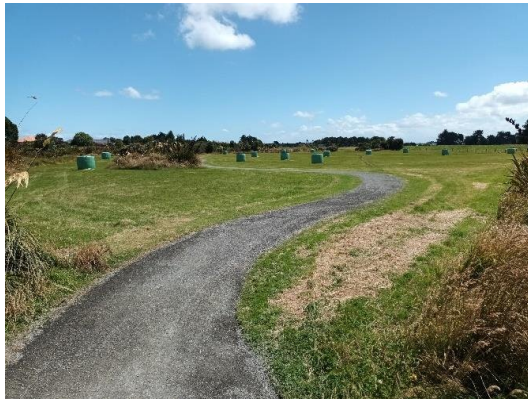
Figure 7: Part of the resurfaced path at Talbot St Reserve.
