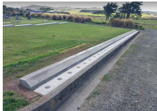
Figure 6: New ash beam at Greenpoint Cemetery.
