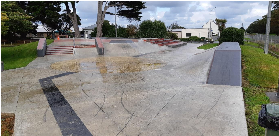
Figure 10: The Elles Road Skate Park after resealing has been completed.
