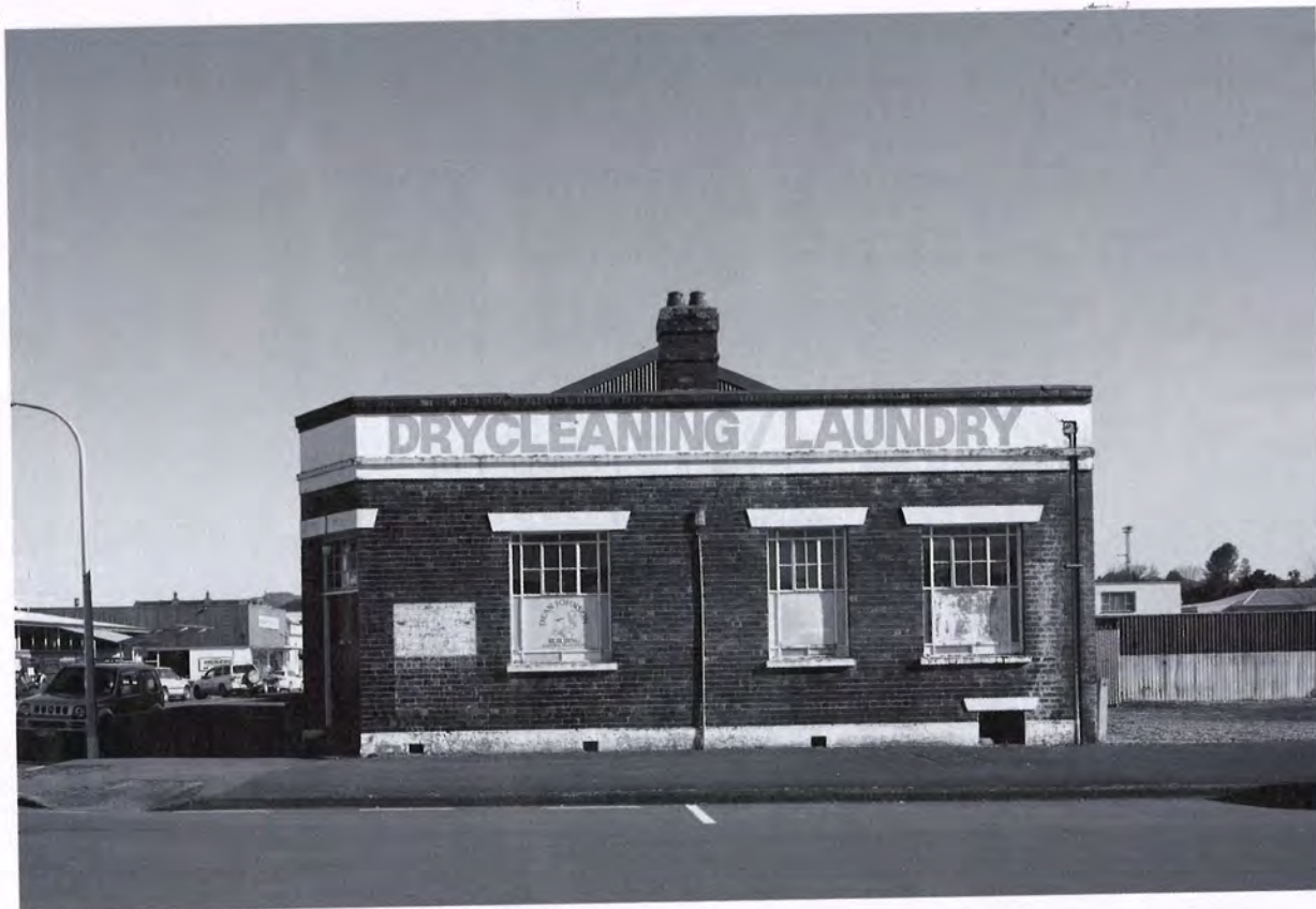
Unreinforced masonry buildings such as the Dean Johnson Building in Taumarunui are a familiar part of small-town and suburban New Zealand.
